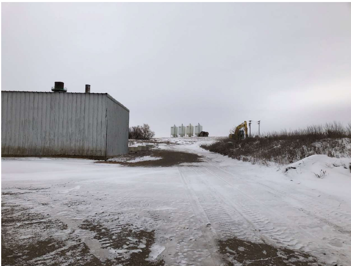
Figure 7 – Gascoyne Materials Handling & Recycling Storage Buildings
