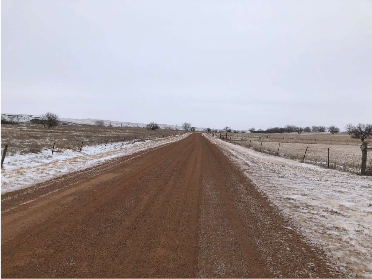
Figure 10 – Lehigh Drive, Stark County Right of Way
