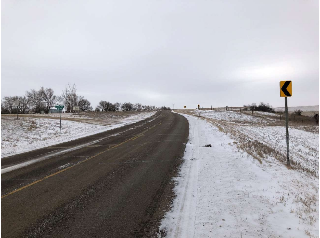
Figure 3 – Lehigh Road and Lehigh Drive Intersection, Stark County Right of Way
