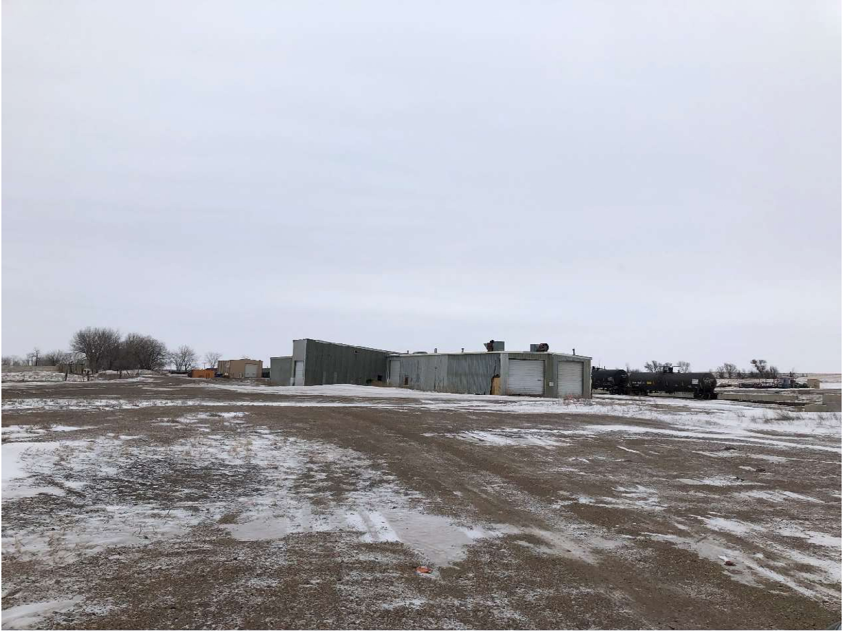
Figure 6 – Gascoyne Materials Handling & Recycling Storage Buildings
