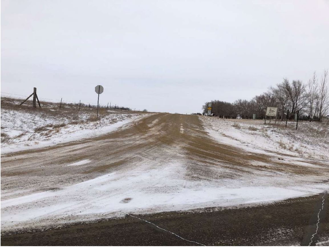
Figure 4 – Lehigh Road and Lehigh Drive Intersection, Stark County Right of Way
