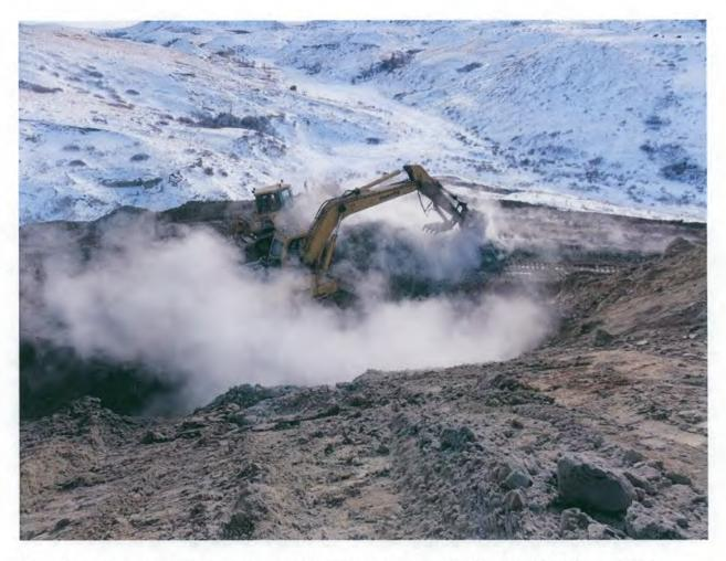
This photo shows work in progress to extinguish the Horseshoe Creek 3 Coal Seam Fire in McKenzie County.
