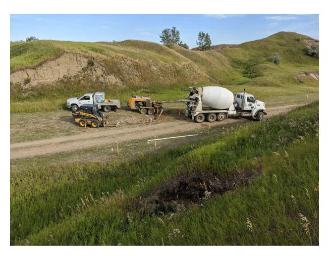
Contractors Use Foamed Sand to Fill Underground Mine Voids
