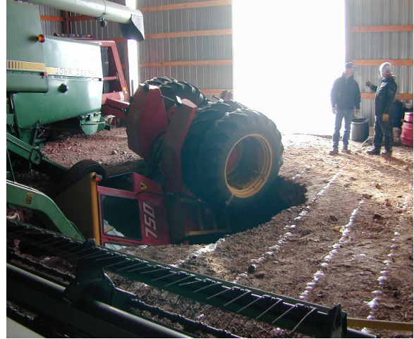
2001 Beulah (Garner Sailer) Emergency, sinkhole inside a machine shed.
