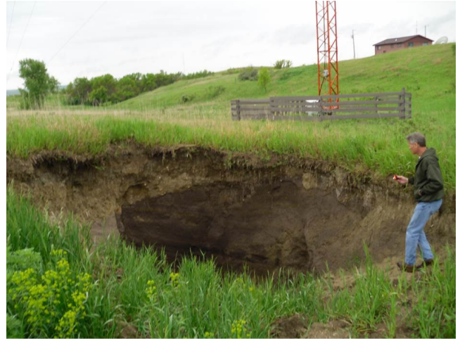
2010 Beulah (KDKT) Emergency, sinkhole near KDKT Radio Tower, Beulah, ND.
