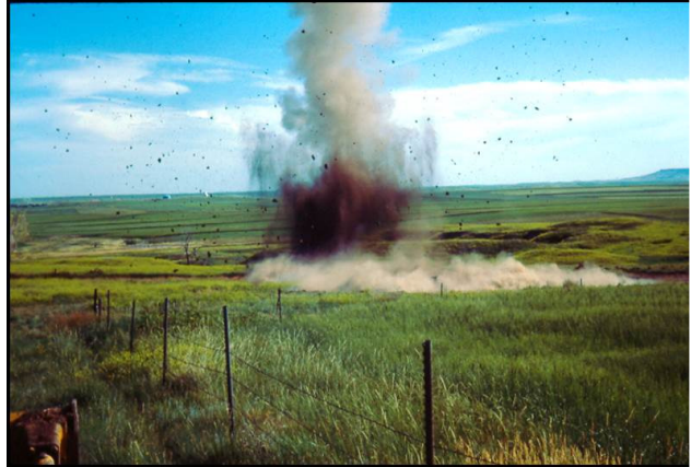
Blasting underground mine at New Leipzig in 1983
