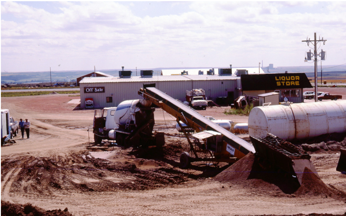
A 1985 slurry-fill drilling and grouting project near Beulah
