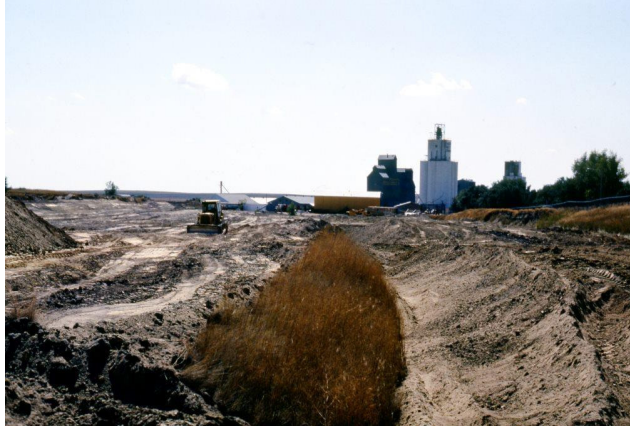
Daylighting underground mine at Scranton in 1983
