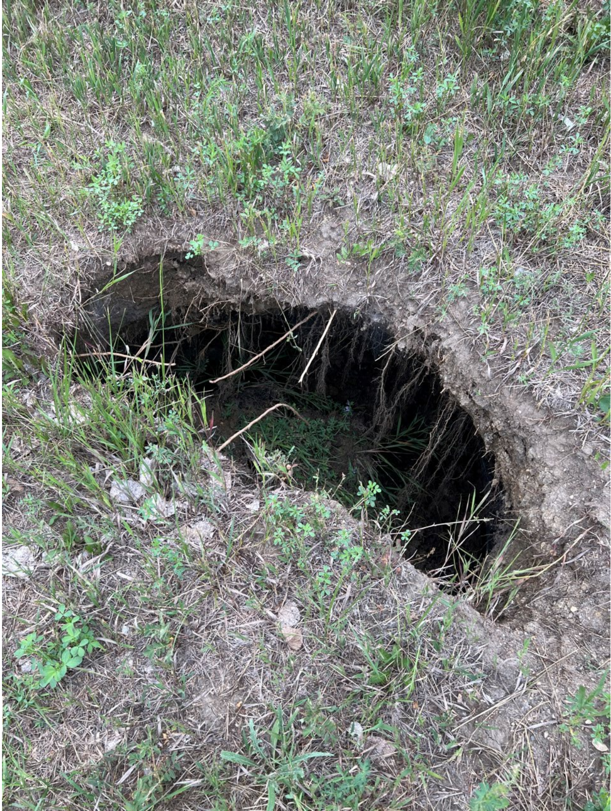
Figure 1: A sinkhole opened up in the McLean County Highway 15 right of way in the spring of 2022.
