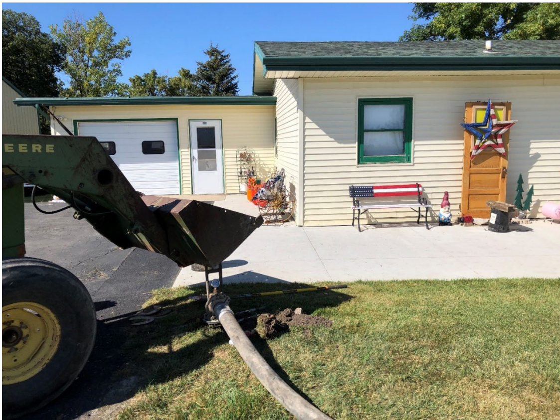
Figure 4: Approximately 60 yards of grout was pumped into this hole.
