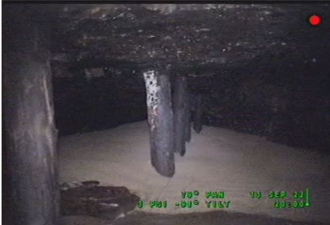
Figure 3: A borehole camera image shows timbers in the mine workings. The tan material is grout slowly filling this portion of the mine.
