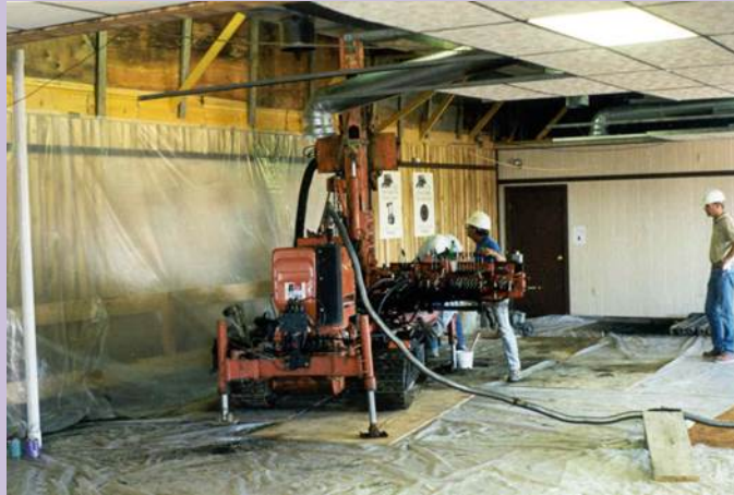
Drilling & grouting inside a building at Beulah, 1997.
