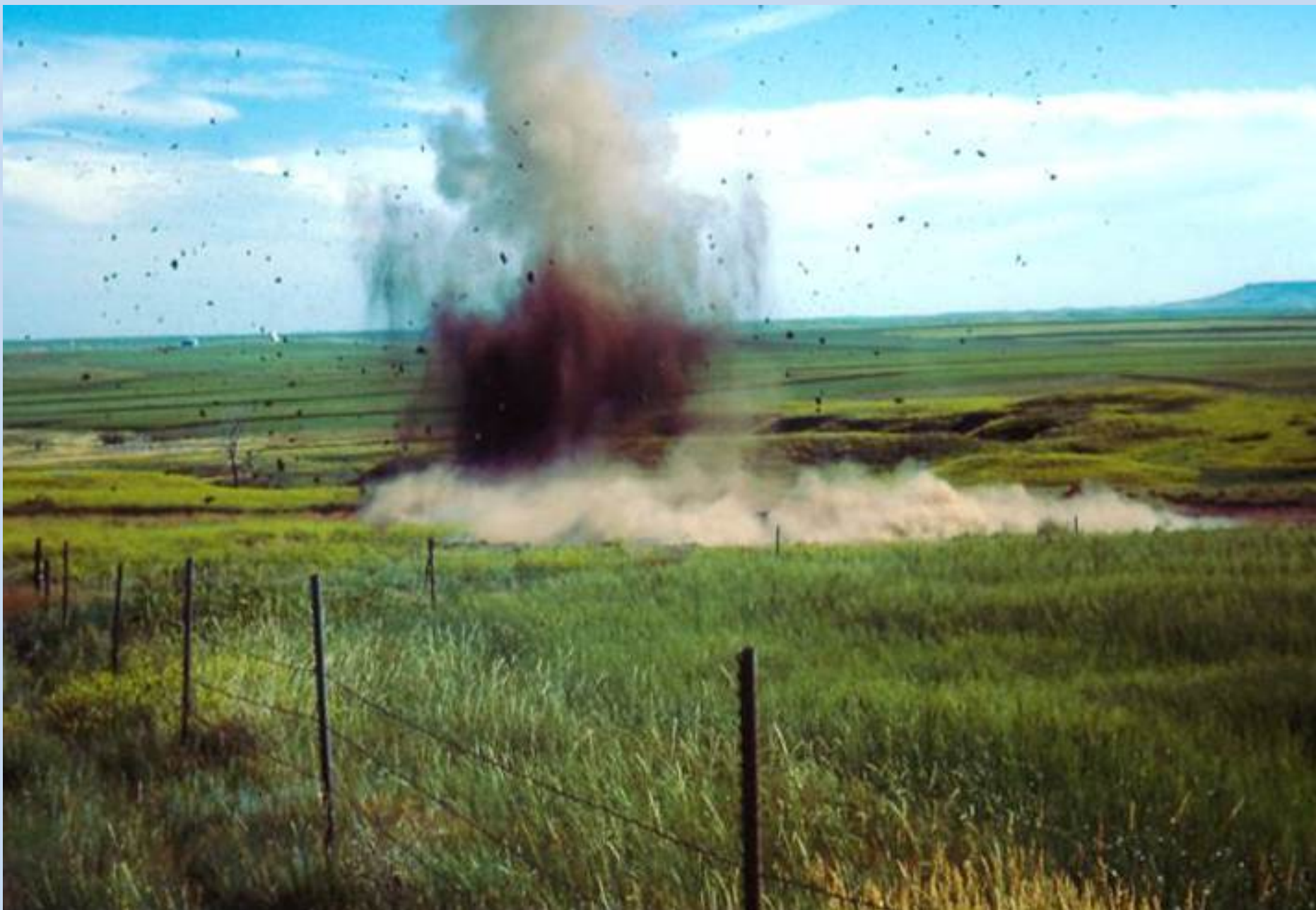
This shows blasting to collapse underground mine workings near New Leipzig, ND, in 1983. This method wasn't very effective and had the potential for adverse consequences.
