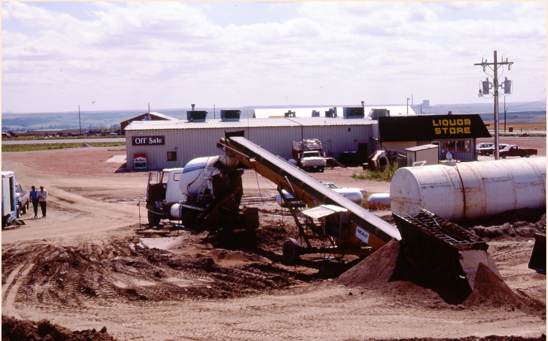
This shows a 1985 slurry-fill drilling and grouting project near Beulah, ND. Three large drilling and grouting slurry projects were conducted between 1983 and 1987 in an attempt to stabilize collapsing underground mine workings beneath a complex of commercial buildings and several highways near Beulah between 1983 and 1987.
