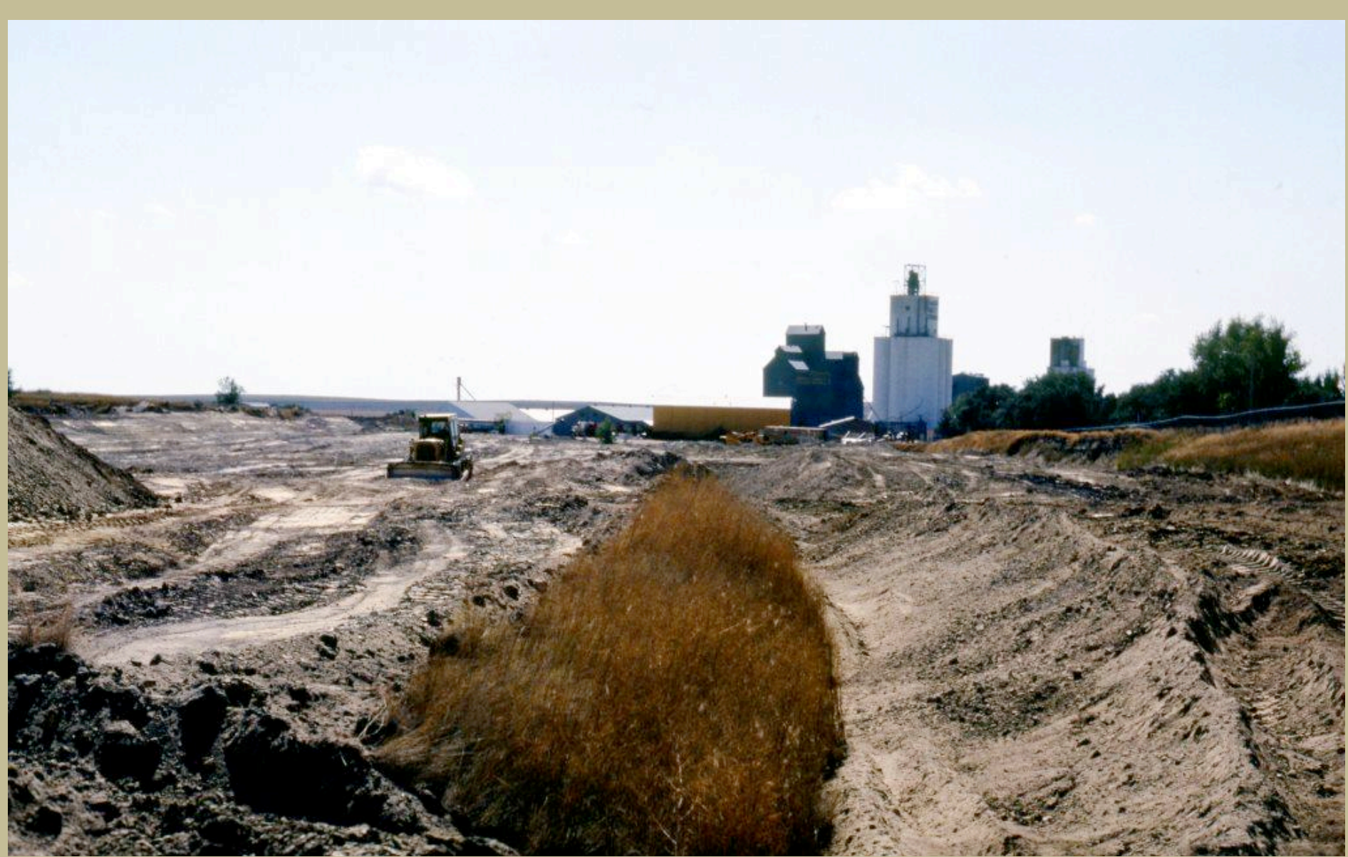
This shows a portion of the daylighting project at Scranton in 1983. Large equipment removed all the soils down to the original mine level, approximately 60-70 feet, and replaced it.
