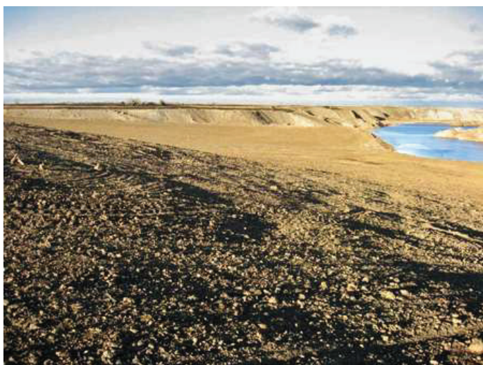
2012 will mark the completion of 14 reclamation projects at the Columbus Mine. These projects were conducted to backfill nearly nine miles of dangerous highwalls and level and revegetate about 700 acres
