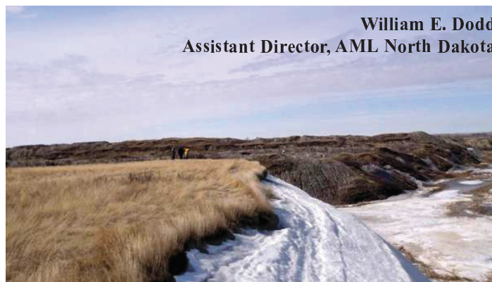
Primary hazards at the Columbus Mine were steep mine highwalls. These nearly vertical cliffs remaining from final pits were 60 feet high in some areas. Other adverse impacts of mining included barren and unstable highwalls, hazardous water bodies and decrepit equipment and facilities.
