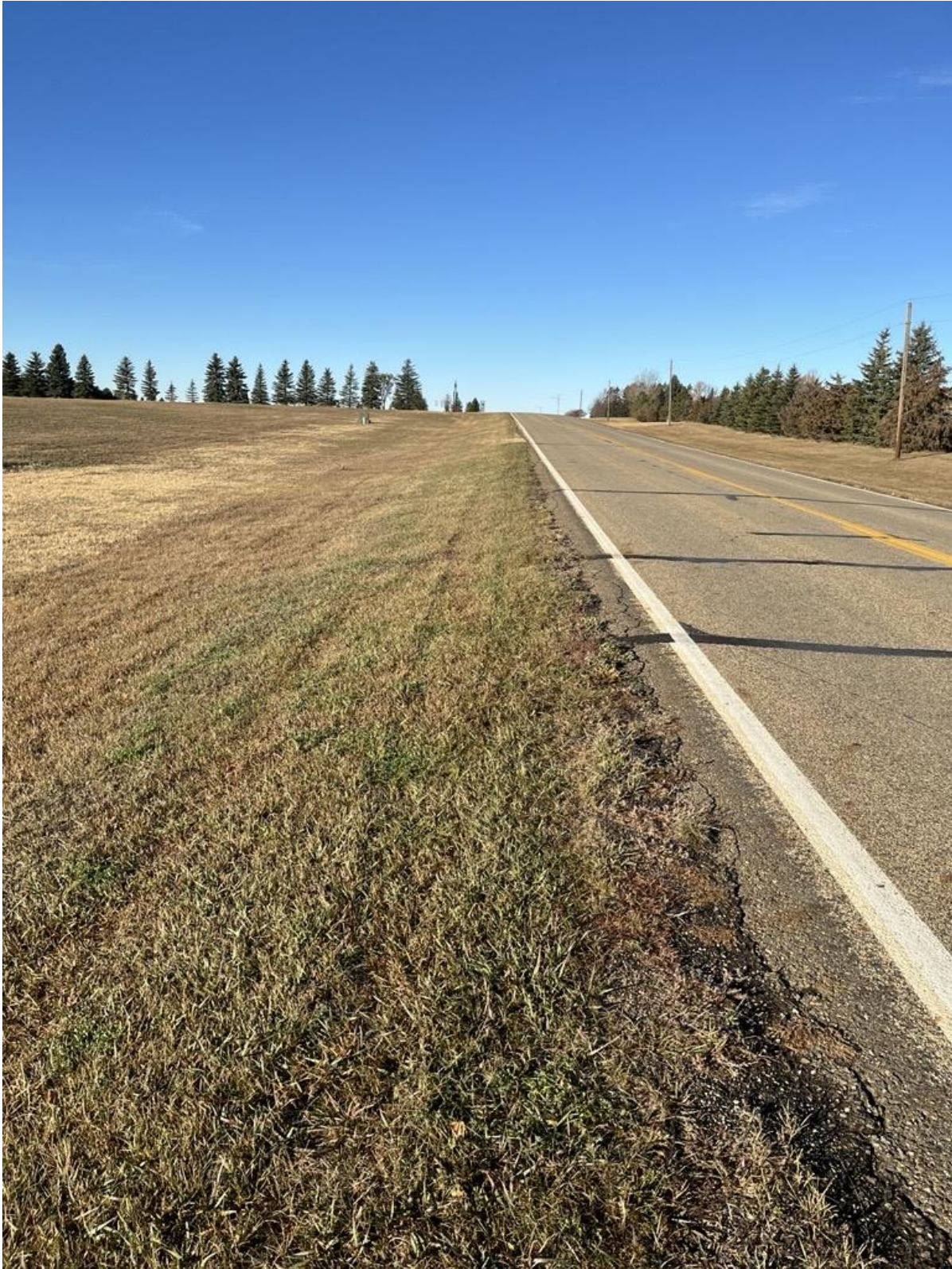
Figure 2 – Ash Ave., Morton County Right of Way
