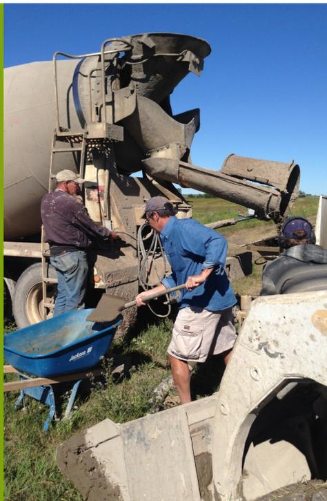
If we have an open void or don't want the grout to travel as far we use a lower slump grout between 6 and 8 inches. Just for comparison, most poured cement has a 1-3 inch slump-very stiff.
