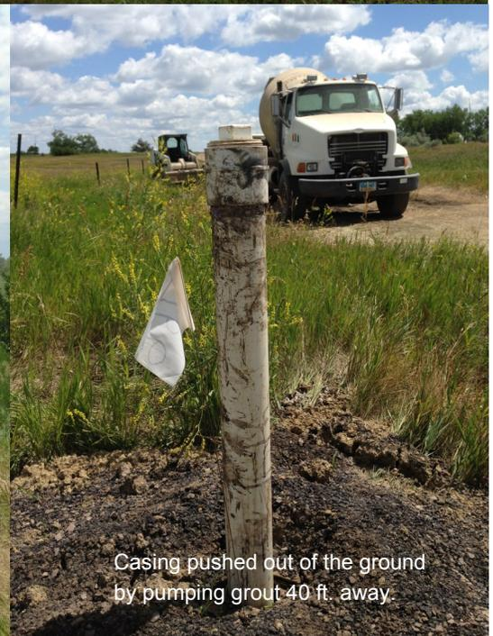
Casing pushed out of the ground by pumping grout 40 ft. away.
