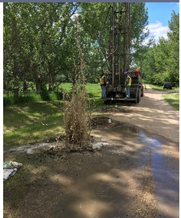
Right: Drilling on 29th Avenue NW in Burlington. Groundwater is being pushed to the surface by drilling 40 feet away. This suggests there may be an opening linking the two holes. Three holes in this area encountered mine workings and were cased for future work.
