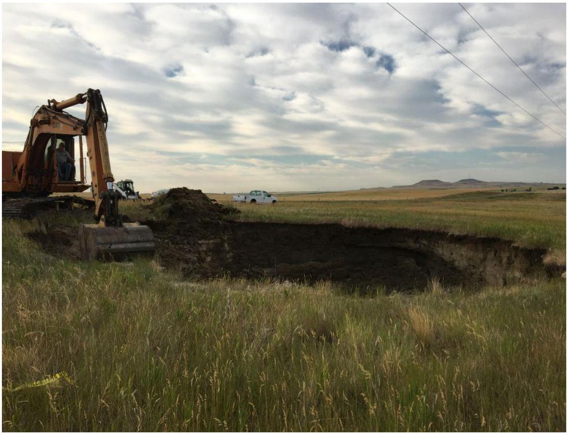
Work began on the 2017-2018 Sinkhole Filling AML Project on July 21, 2017, about 4 miles north of Bowman. This sinkhole was about 30 feet long, 20 feet wide and 18 feet deep. It was located on property owned by the City of Bowman (see cover photo).
