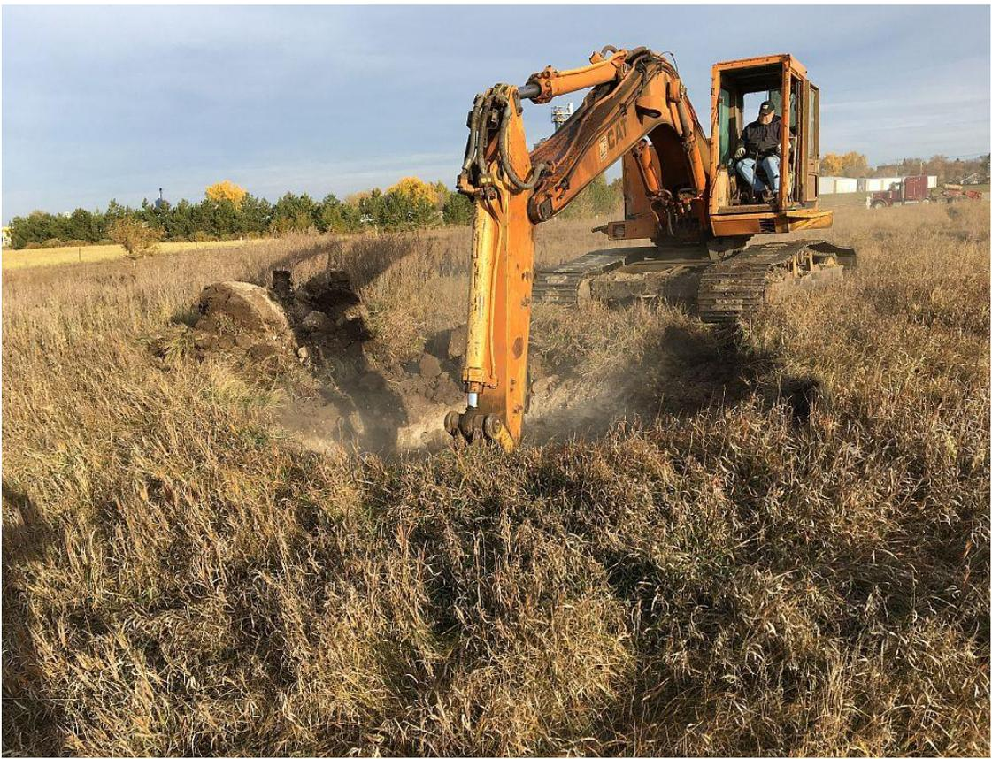
This shows the excavation of a sinkhole south of Garrison. It was about 8 feet in diameter and 10 feet deep. Thirteen sinkholes were filled at this site on October 19, 2017, and the contract cost for this work was \$1995.
