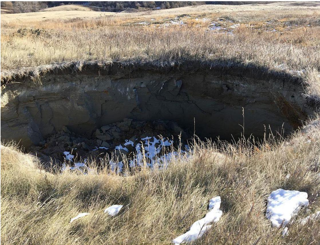
This was a typical sinkhole on North Dakota Game & Fish property, north of Beulah. It was twenty feet in diameter and fifteen feet deep, and more than ten scraper loads of dirt were needed to fill it.
