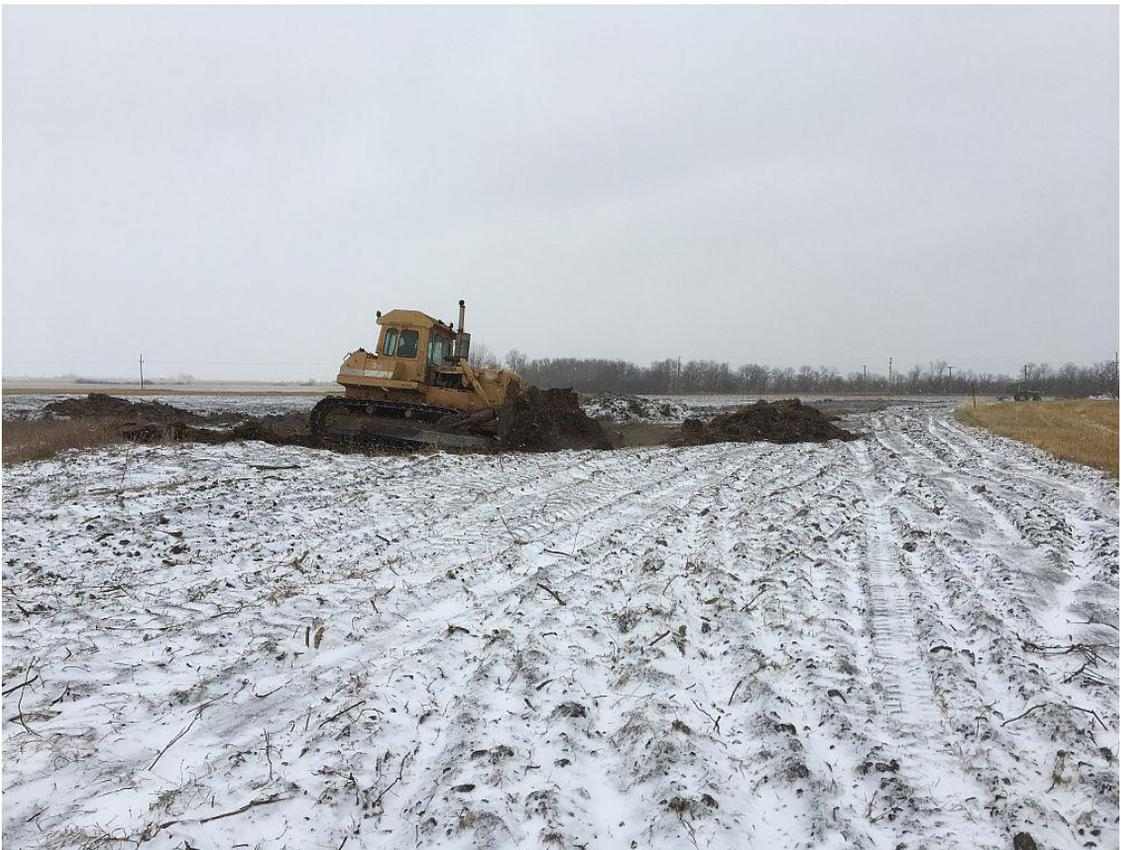
This shows the contractor saving topsoil from around a sinkhole during a snowstorm on November 3. Approximately 1000 cubic yards of dirt were moved to fill the 31 sinkholes at a cost of \$9750.
