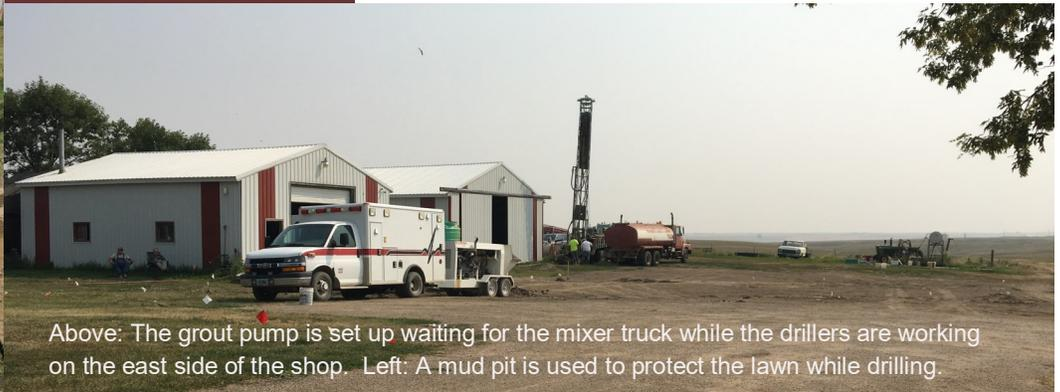
Above: The grout pump is set up waiting for the mixer truck while the drillers are working on the east side of the shop. Left: A mud pit is used to protect the lawn while drilling.
