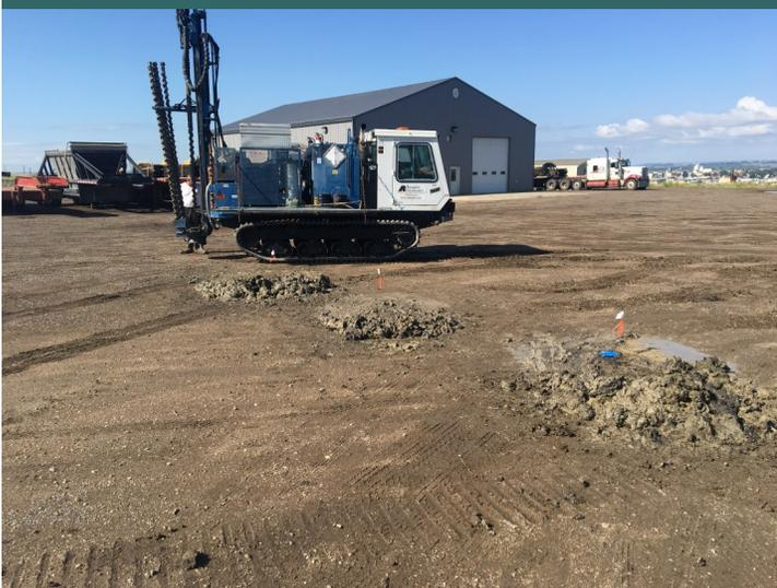
This drill rig ready to begin drilling a new hole. Piles of cuttings show the locations of recently drilled holes.
