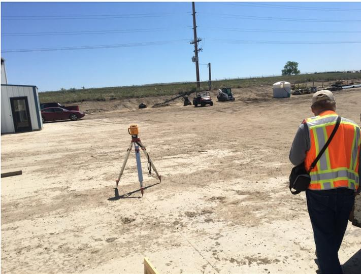
A laser level monitors ground movement near the Shirt Services building during grout pumping. Inspector, James Thornburg, is on the right.
