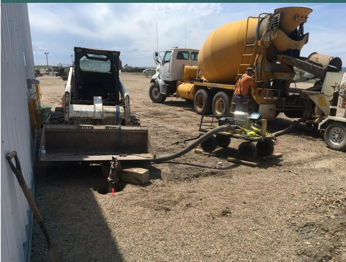
The grout runs through the meter to monitor the pressure. It then goes into the cased hole right next to a building.
