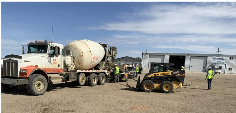
A Knife River truck lined up to pump grout in the Shift Services lot in Williston. Each truck holds 9 cubic yards of grout.
