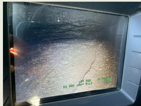
Left: A view from the monitor of the borehole camera: The camera is suspended above the void and recording the foamed sand as it flows into a void.
