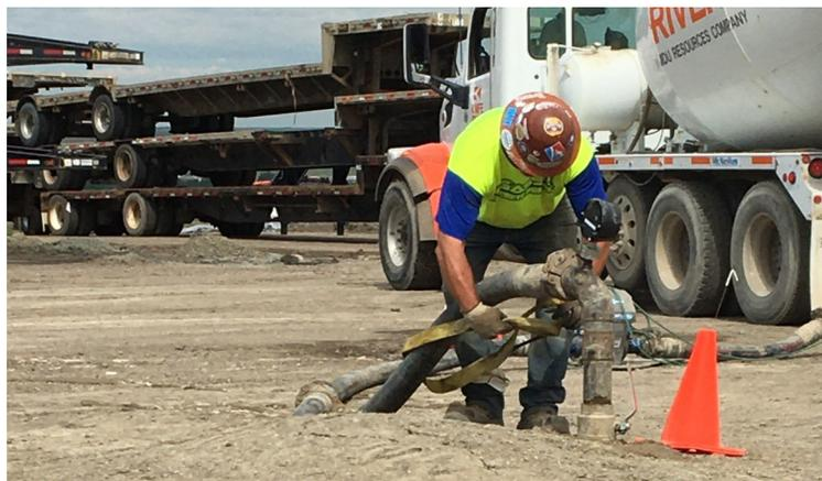
Above: Eric Wagner, owner of Agassiz Concrete Pumping, detaching the pump from a cased hole at Williston.
