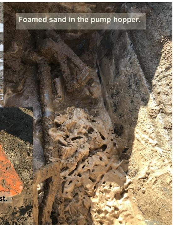
Foamed sand in the pump hopper.
