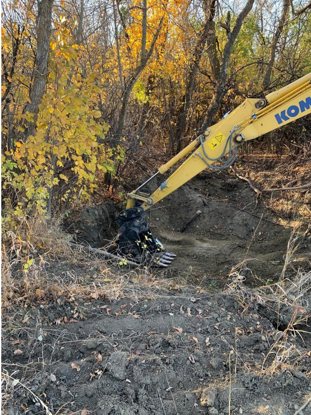
**Figure 9:** This sinkhole is being compacted and graded with an excavator.
