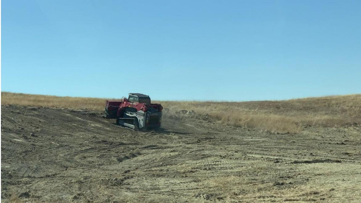
**Figure 4:** A skid steer with a till attachment was used to till the reclaimed sinkhole areas.
