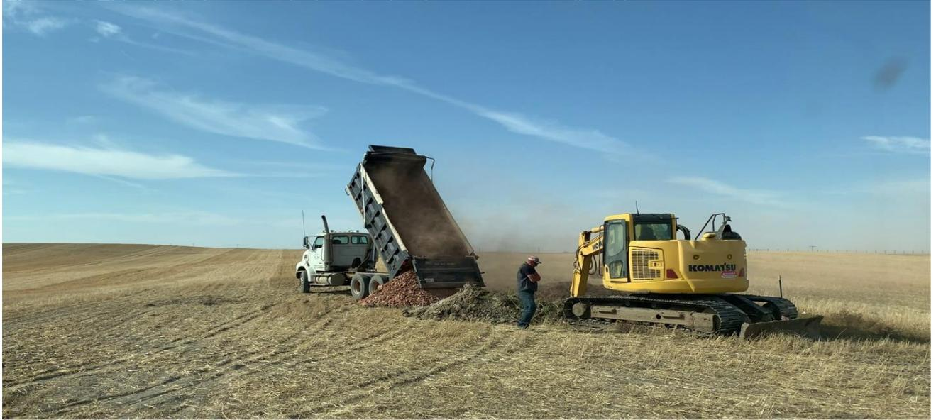
**Figure 6:** This sinkhole is being filled with scoria and soil from a nearby borrow location provided by the landowner.
