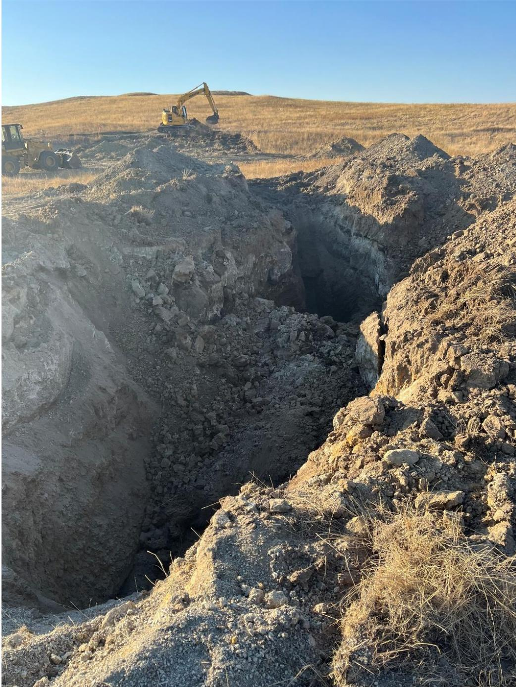
**Figure 3:** This mine void tunneled extensively underneath the ground's surface.
