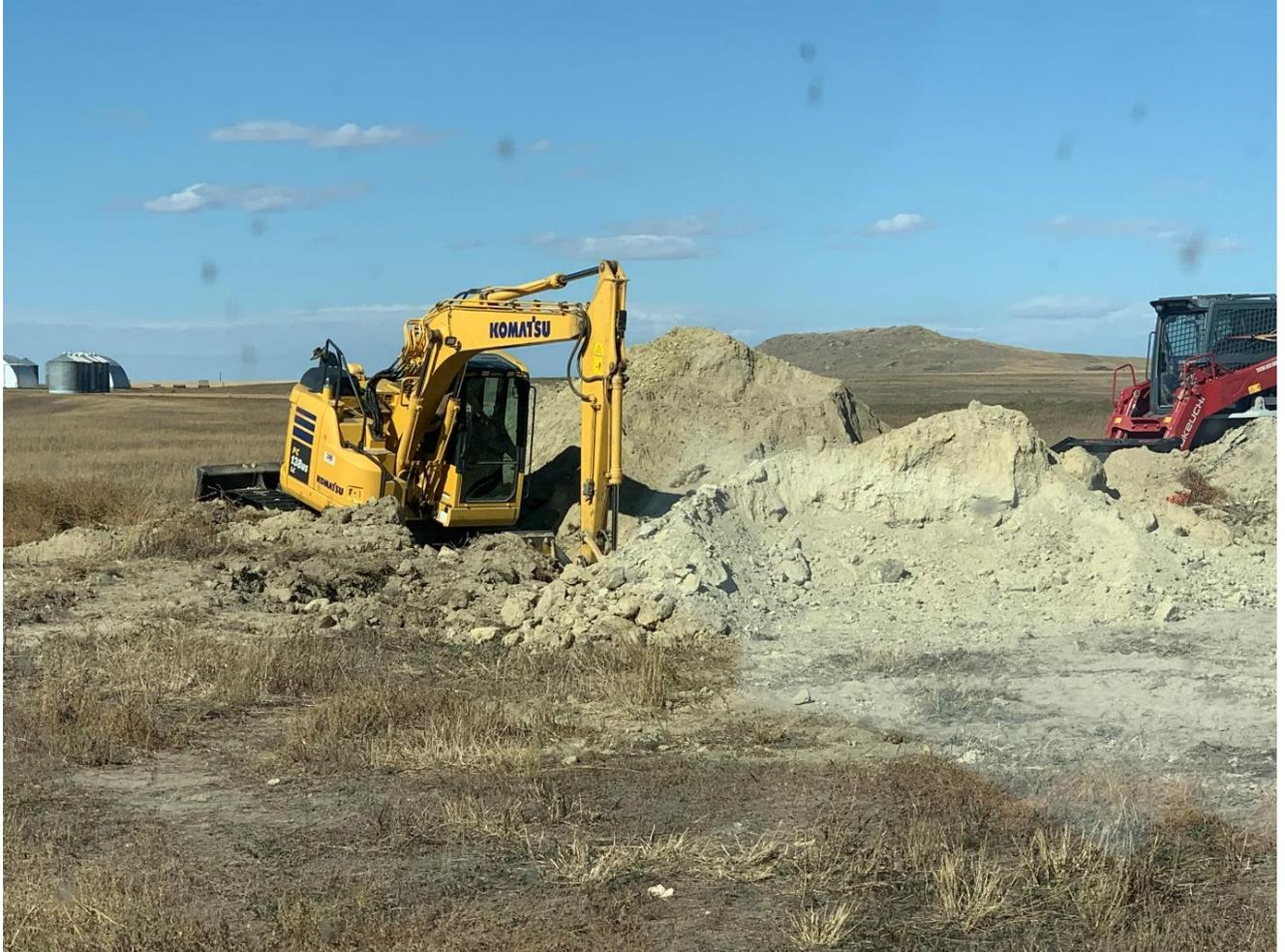
**Figure 2:** When the excavator opened up this sinkhole, the mine void was more than twice as large as expected.
