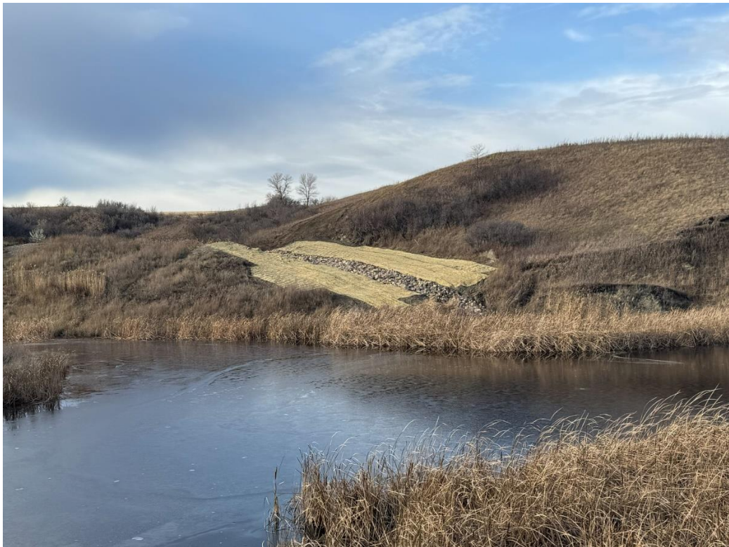
Figure 12: A rock channel was installed to replace a culvert with unstable, eroding soil.
