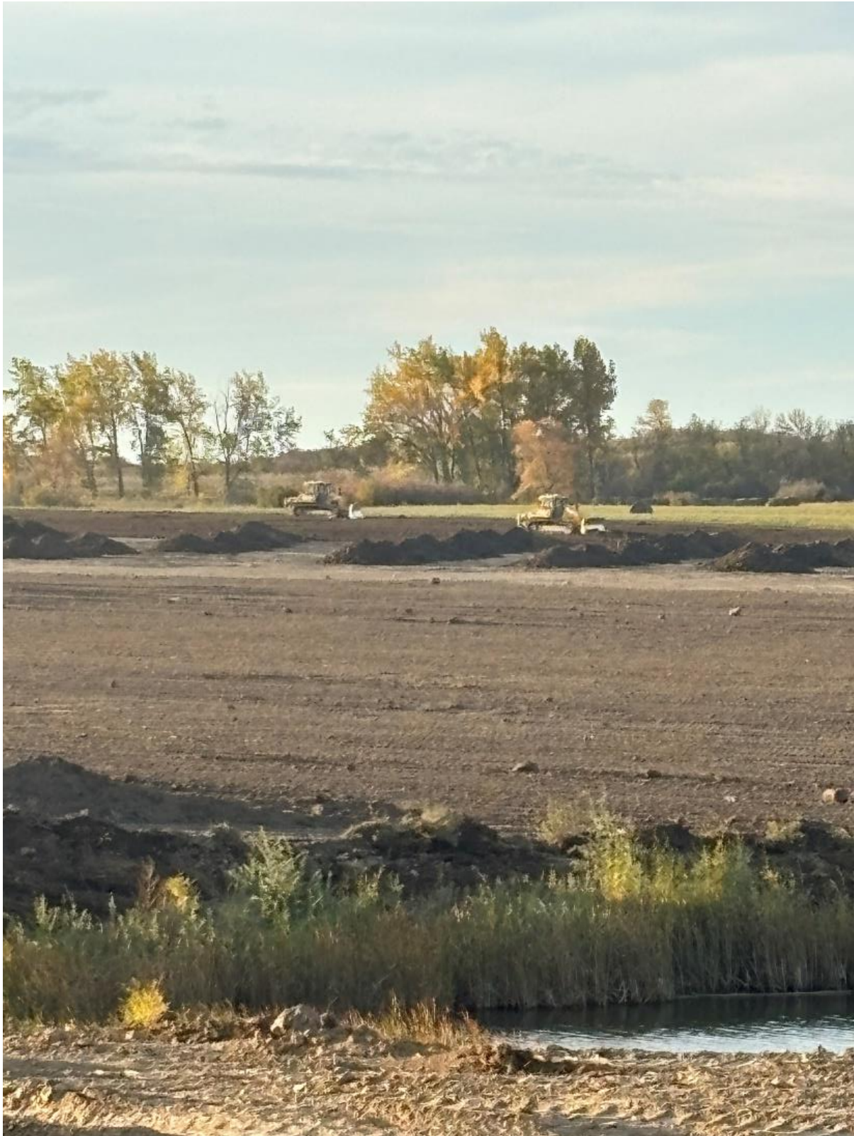
Figure 7: Dozers are respreading topsoil.
