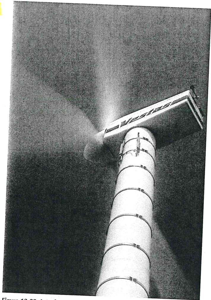
Figure 13-23. Interference, no; ugly, yes. Vestas V47 with awkward telecom antennas in Germany. While the wind turbine is obviously not interfering with telecommunications here, the antennas and their mounting hardware give this Vestas turbine an undesirable industrial appearance.
