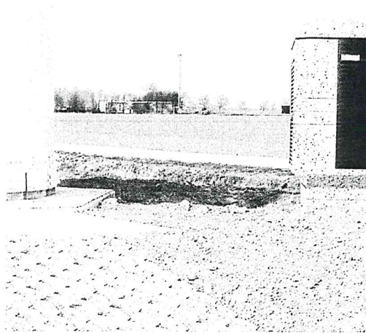
Figure 13-16. Architectural transformer treatment. Where transformers cannot be placed inside the tower, transformers should be shrouded with an architectural treatment. The transformer on the right incorporates a facade to harmonize what otherwise would be an industrial structure with other nearby structures on the landscape. Open-cell concrete pavers harden the access track to the NEG-Micon tower on the left, allowing rain to percolate through to the groundwater table. This turbine and the Lagerwey 18/80 in the background are owned and operated by Noud de Schutter, a Dutch farmer in the Wieringemeer polder north of Amsterdam.
