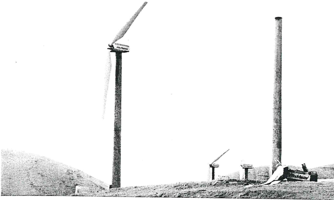
Figure 13-11. Headless horsemen. Dead and dying Windmaster turbines on a wind farm in California's Altamont Pass. When wind turbines are no longer "used and useful," they and their supporting infrastructure should be promptly removed.
