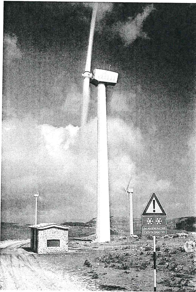
Figure 13-8. Watch for ice. This sign at the Acqua Spruzza test site in Italy's Apennine Mountains warns, WIND TURBINE, WATCH FOR ICE. Europeans typically urge caution around wind turbines, but seldom exclude the public. In this case falling ice could be a hazard, but only during winter storms when few people are likely to visit the windswept site. Note that the roof and facade of the control building are constructed of native materials as used on similar structures elsewhere in this region.
