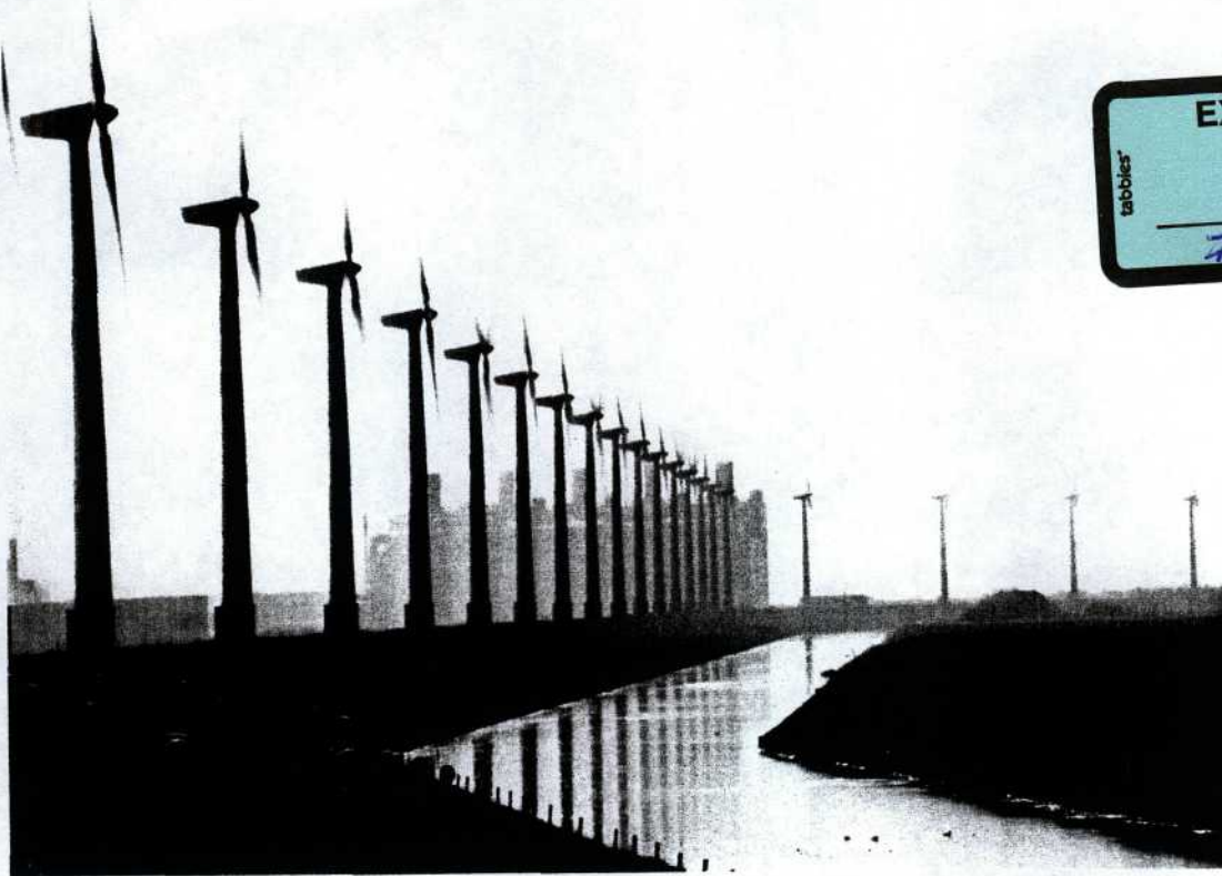
Figure 2-6. Wind power plant. A linear array of modern wind turbines along a canal in the Netherlands. The wind turbines supply bulk electricity to the utility network served by the giant gas-fired power plant in the background.
