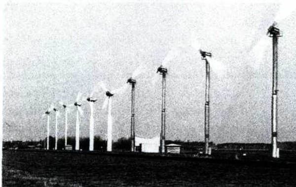
Kennemerwind. The four Lagerwey turbines (right) along the Noord Holland Kanaal are part of the Kennemerwind co-op. Each turbine generates 150,000 to 200,000 kWh per year.
