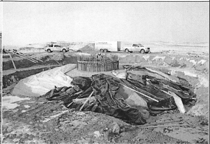
Foundation completely secured for winter
