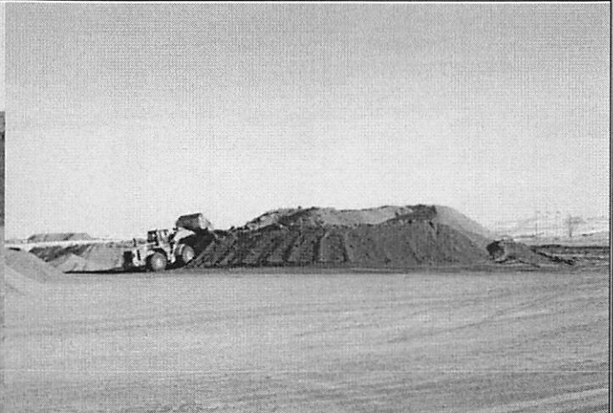
Foundation starting to receive cover for winter
