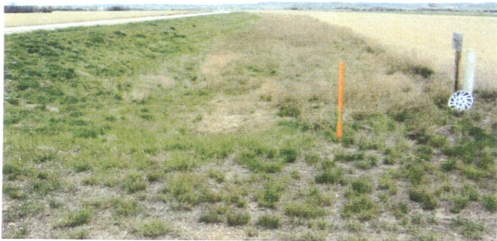
Figure 6: View to the north over corridor route avoiding Fort Buford site area by employing Highway 58 right-of-way (Img. 8-7).
