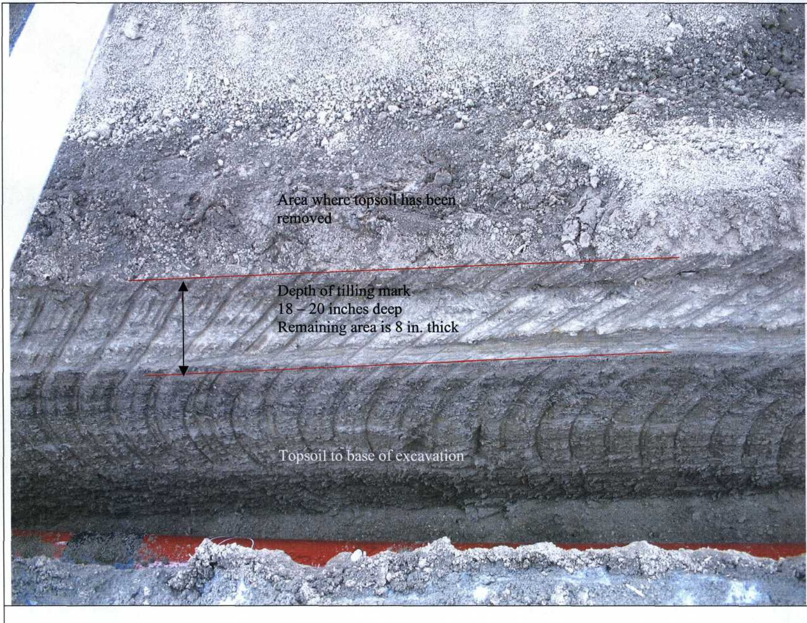
Picture of Topsoil Strata on South end of Section 20 near the railroad tracks
