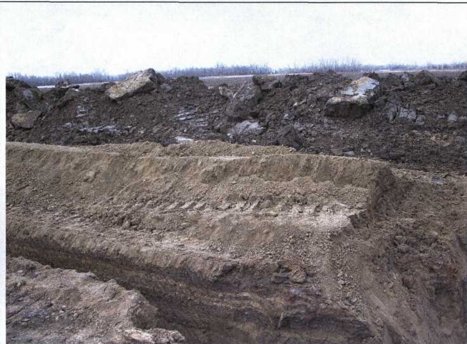
2 S16 east of Missouri River -- east end looking north across ROW
