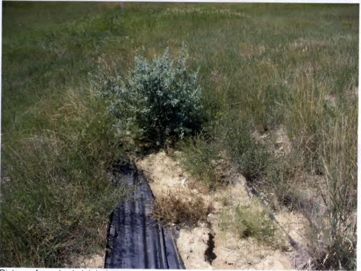
Picture of repaired sink hole
