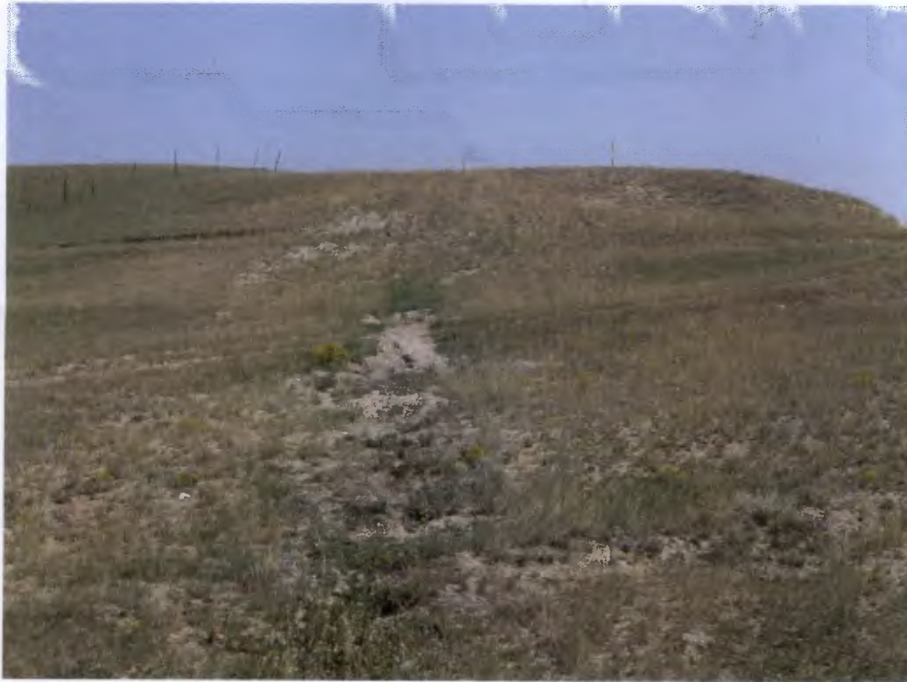
Area on hill where sparse growth area was replanted In foreground – washout that was repaired last year is intact.
