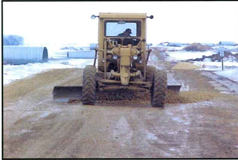
Preparing the Roads
