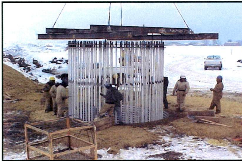
Lowering the Bolt Cage
