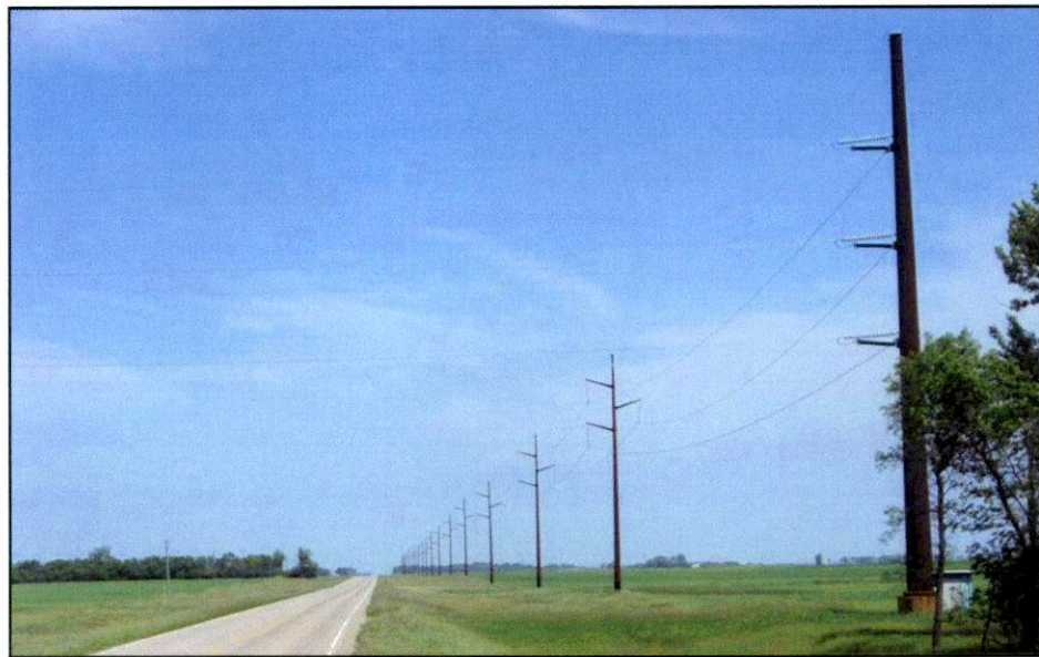
Example of Line Installed Along Right of Way
