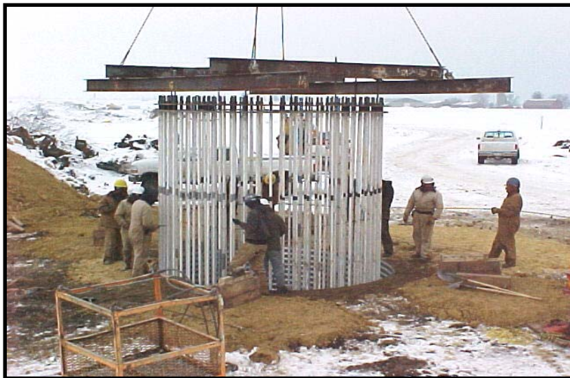
Lowering the Bolt Cage
