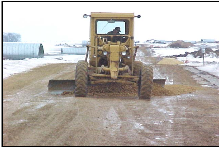
Preparing the Roads
