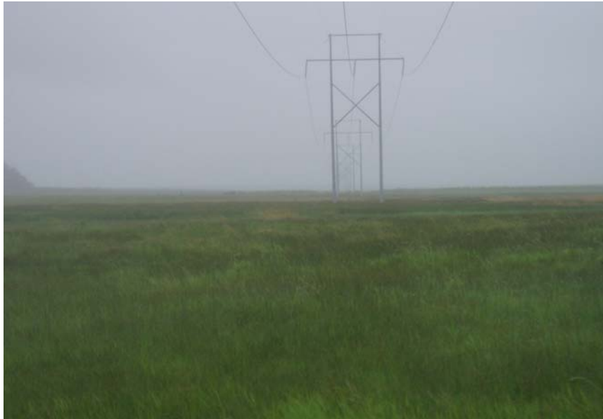
Photo 9: Section 33, Torgerson Township. View to north along existing transmission line. First visible existing structures are in the wetland.
