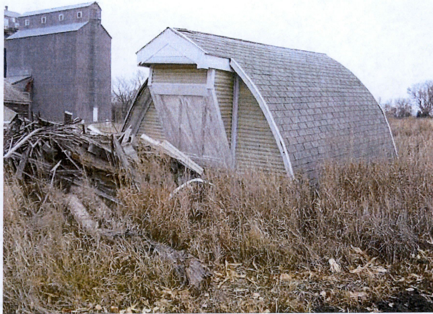
3. Looking north – View of Building 3 (technically a roof of a building).
