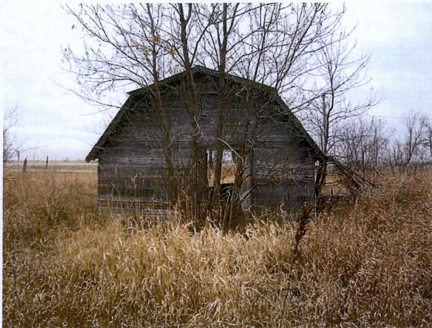
4. Looking west – View of Building 4 (a “storage garage”).
