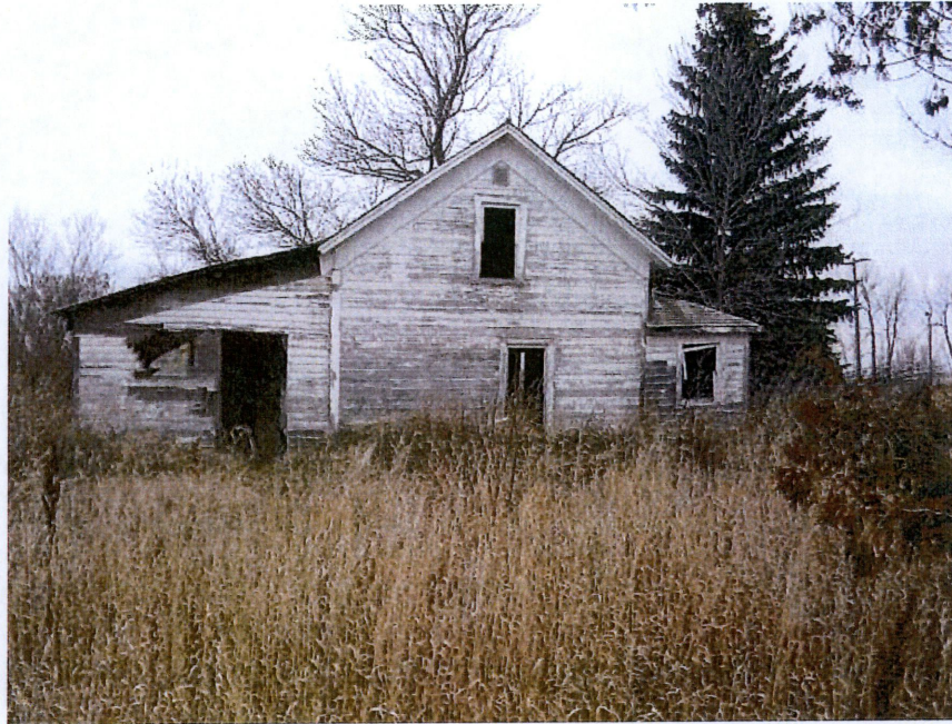
5. Looking east – View of Building 5.
