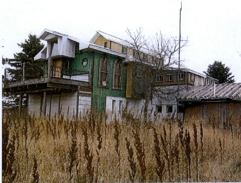
1. Looking east – View of Building 1.
