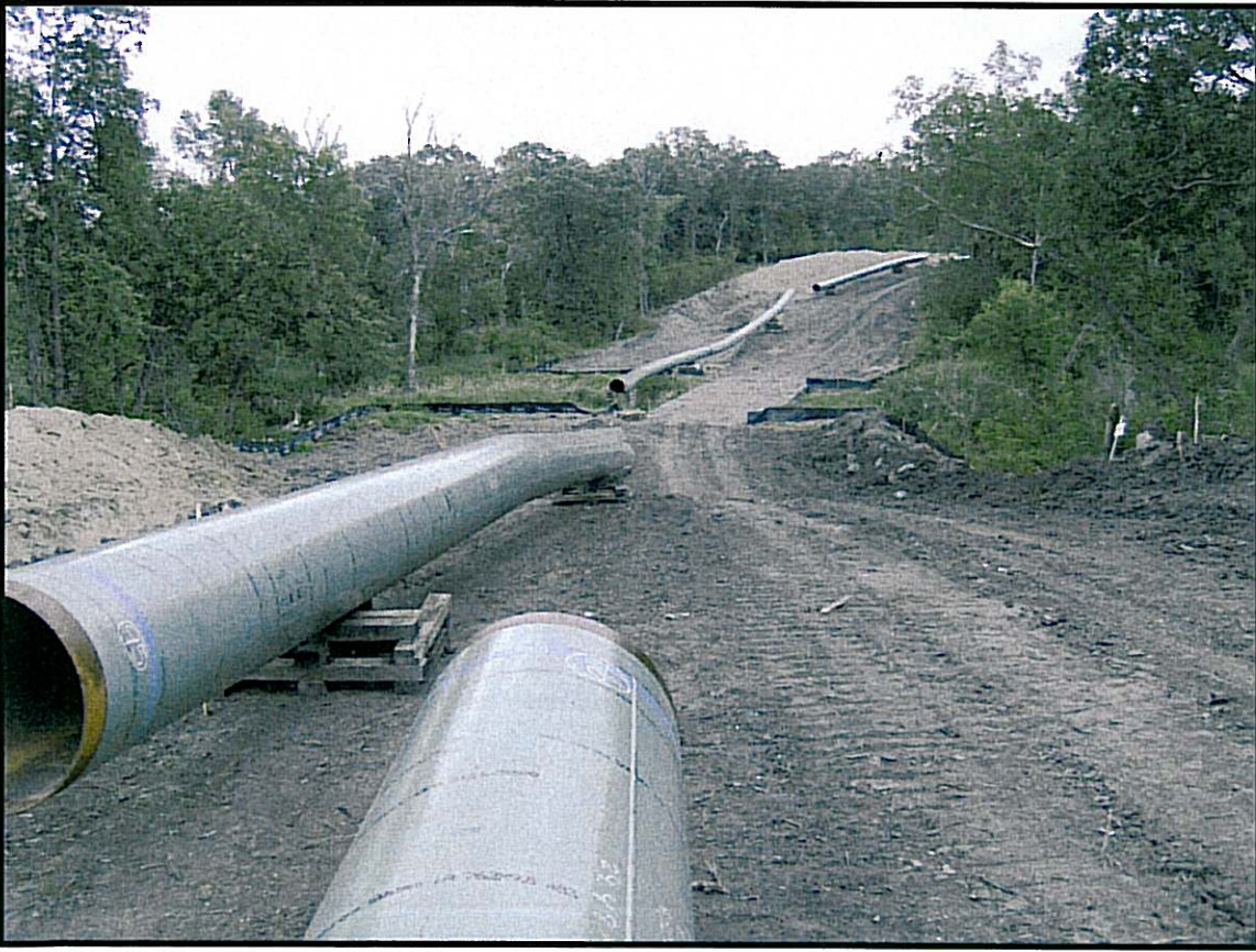
MP 31.8 SWP1NDPE001 View Looking South
