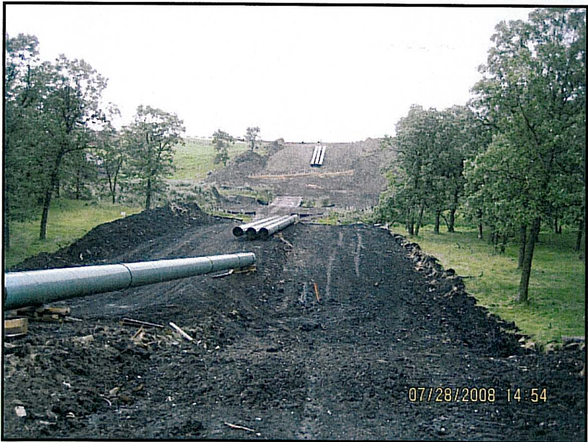
MP 46.5 North Branch Forest River View Looking North
