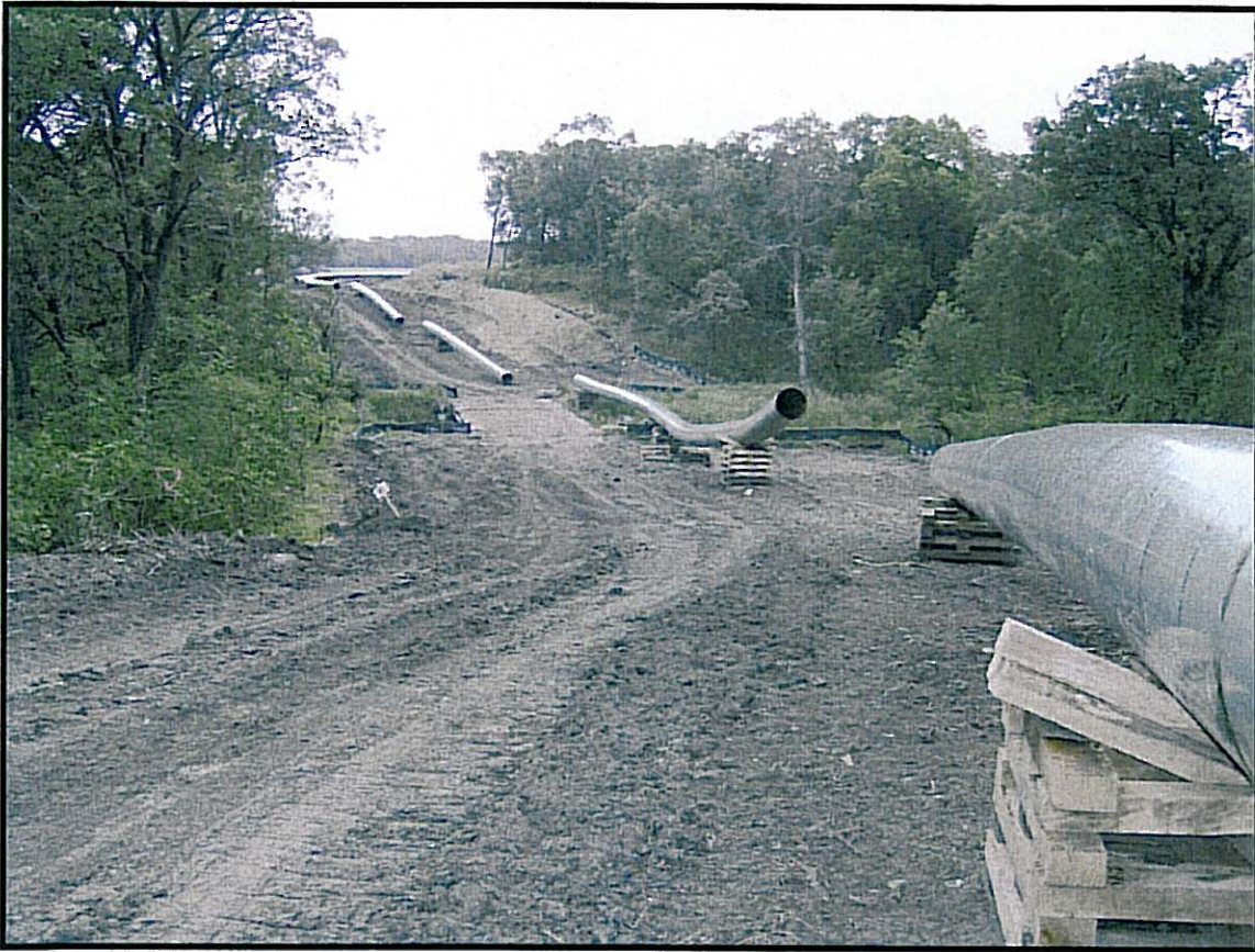
MP 31.8 SWP1NDPE001 View Looking North
