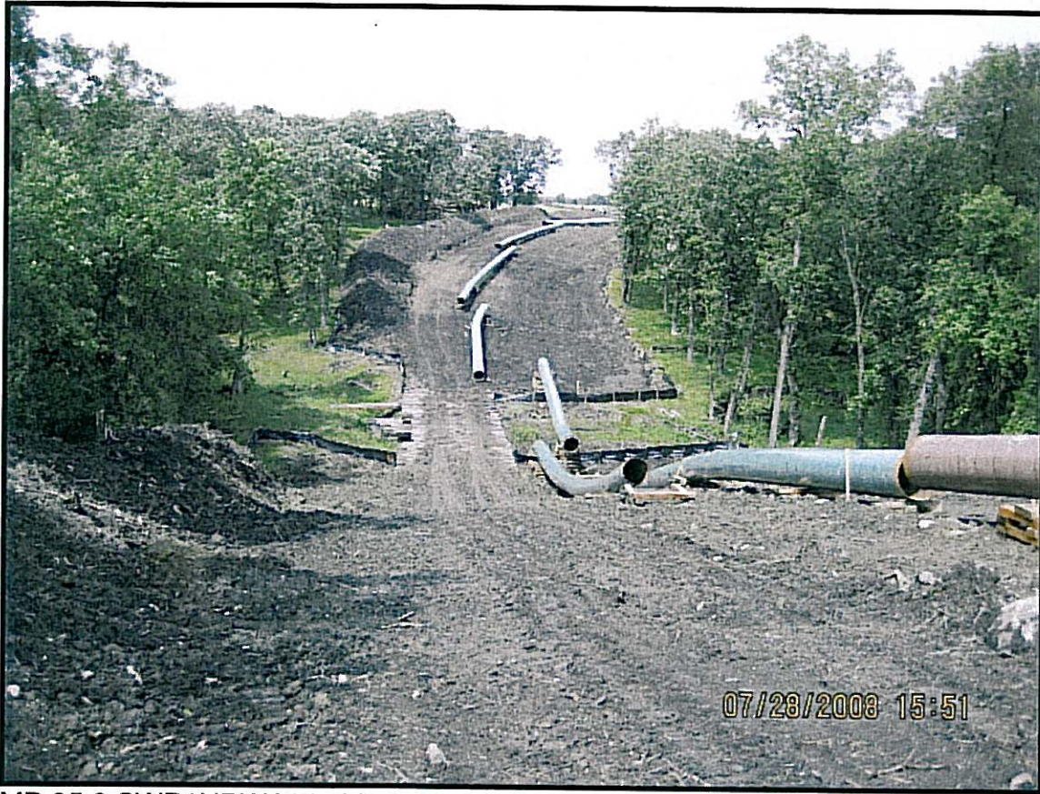
MP 35.3 SWP1NDWA010 View to the North
