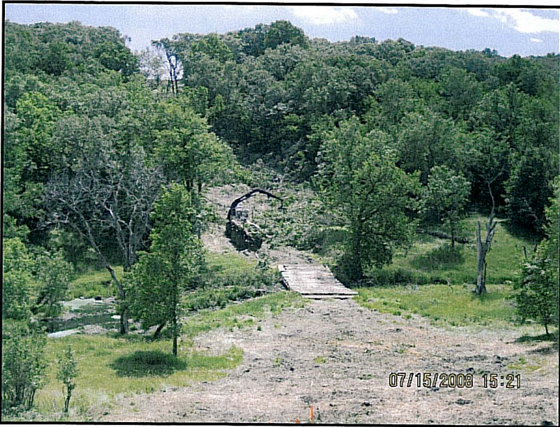
MP 54.8 Middle Branch Forest River View Looking North
