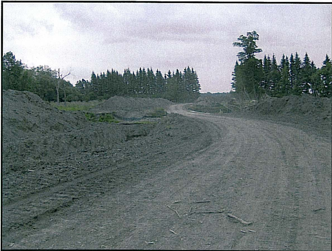
MP 29.5 North Branch Park River (SSC4NDPE201) View Looking South
