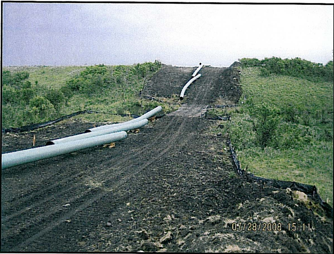
MP 42.7 S_UTM14_0404 View Looking South
