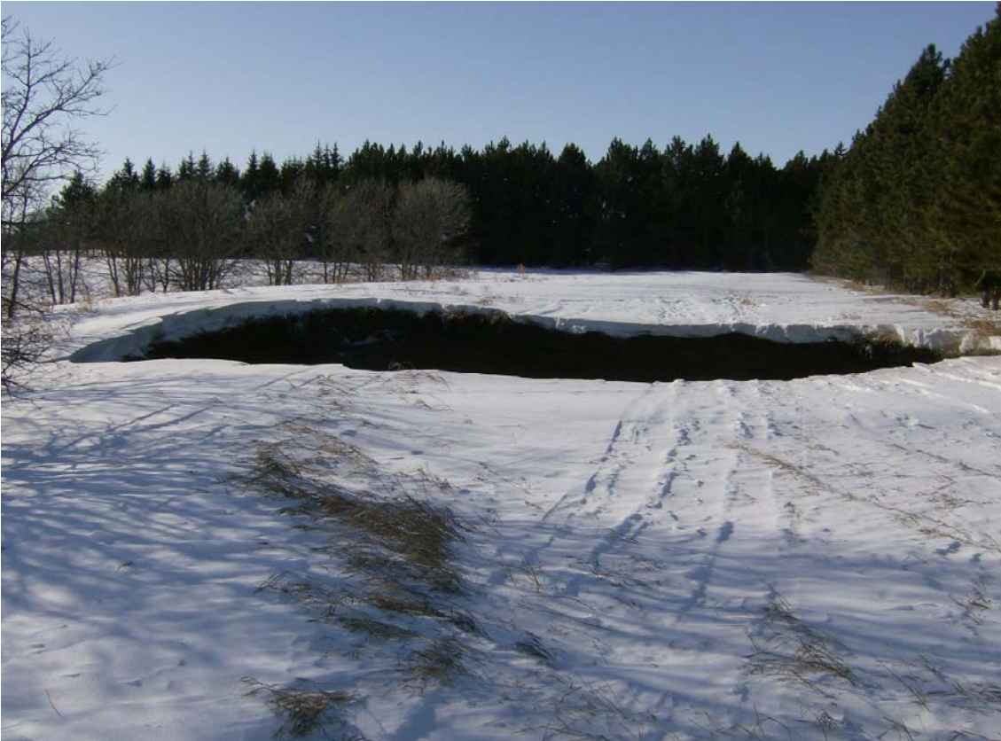
SN 363+00 looking W, Sinkhole near ROW centerline across Tetrault SF overlook road 2009-01-29
