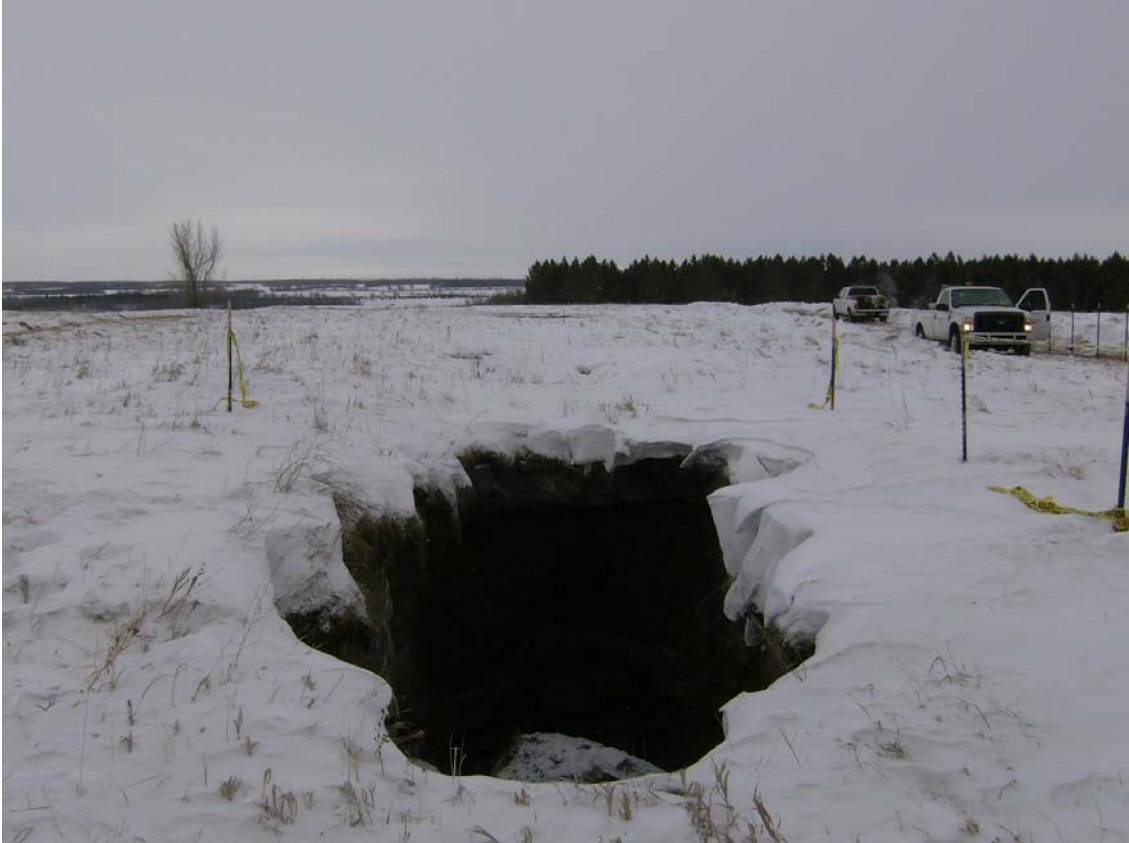
SN 356+15 Sink hole looking south
