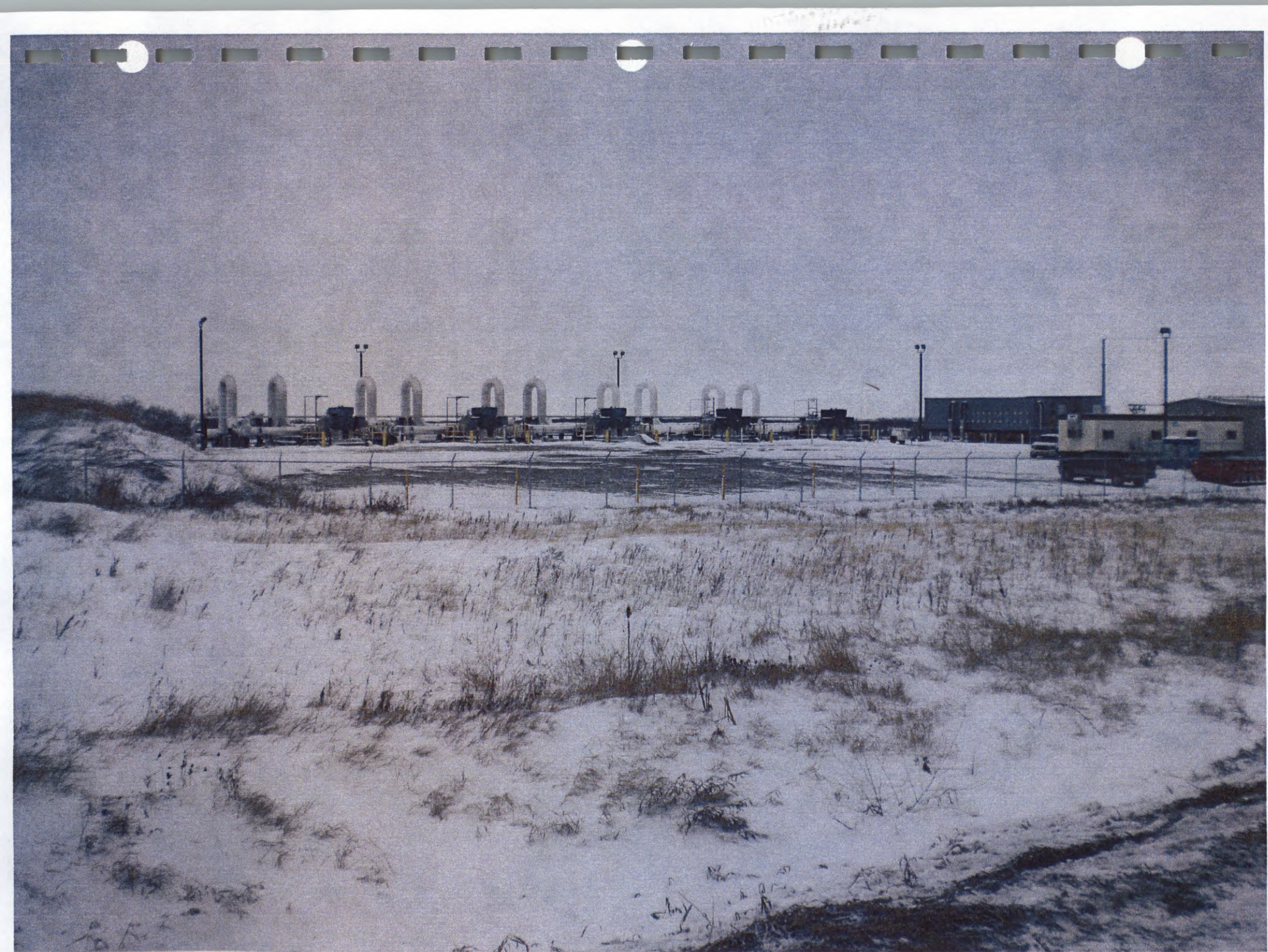
Picture # 33 1st Pump Station 76th St & 126th Ave NE
