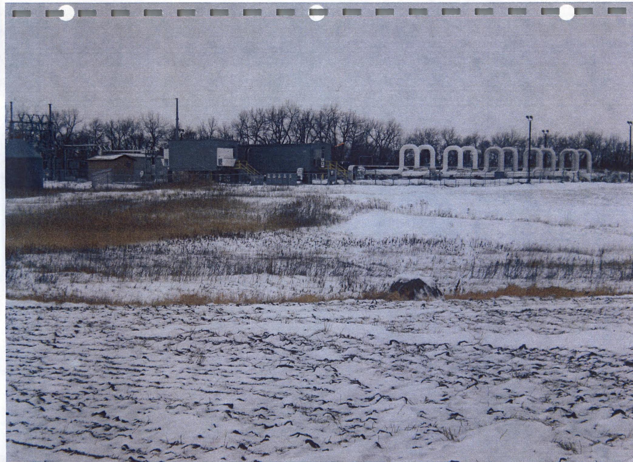
Picture #34 1st Pump Station
