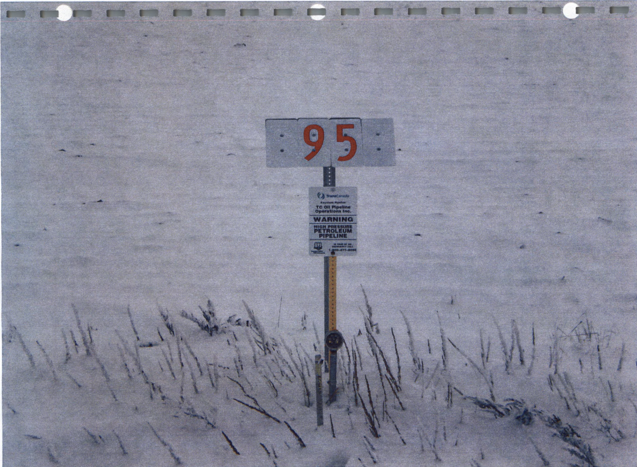
Picture #.50 mm 95 for Air Survey 17 th St/NE Notice Cap missing
