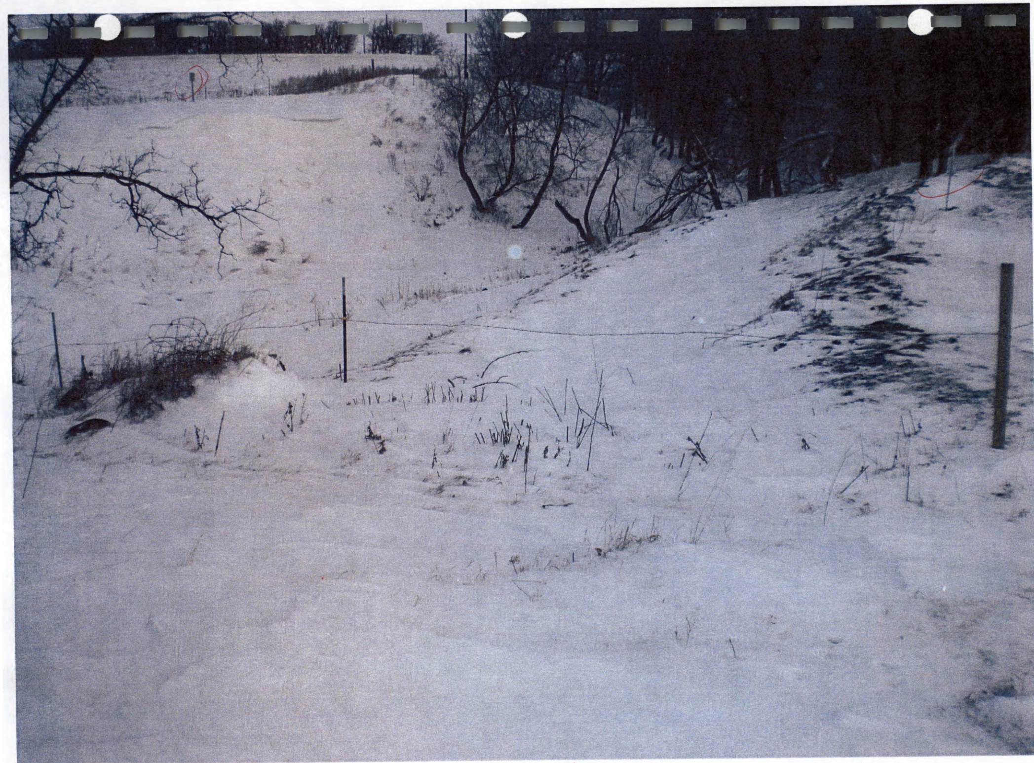
Picture #10 Embankment Terraced, noticed signs on both sides
