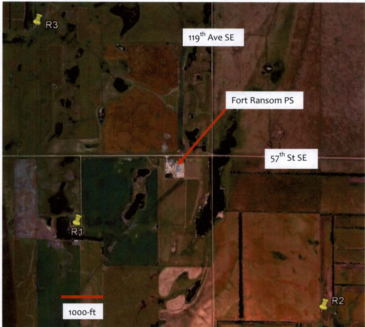
Figure 1: Aerial View of Fort Ransom Pump Station Site and Receptor Locations (R1-R3)
