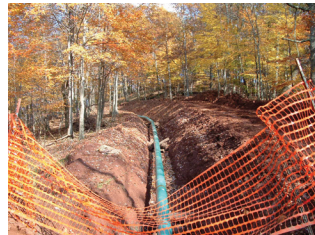
Pipeline in trench
