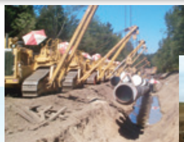
Inspection and repair of coating
