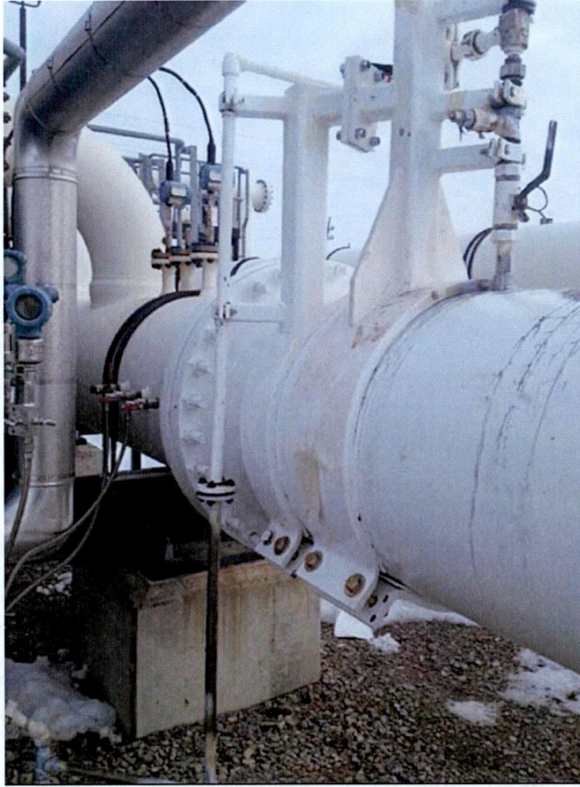
Figure 7: PSV-2206 assembly relocated to piping not exposed to vibration.
