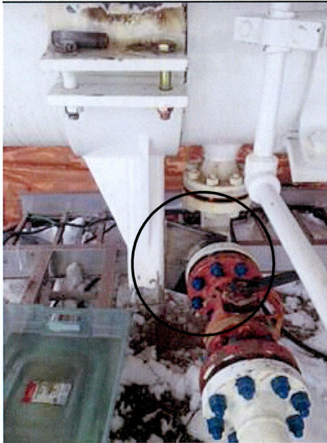
Figure 5: Improved bracing of drain upstream from the PCV.
