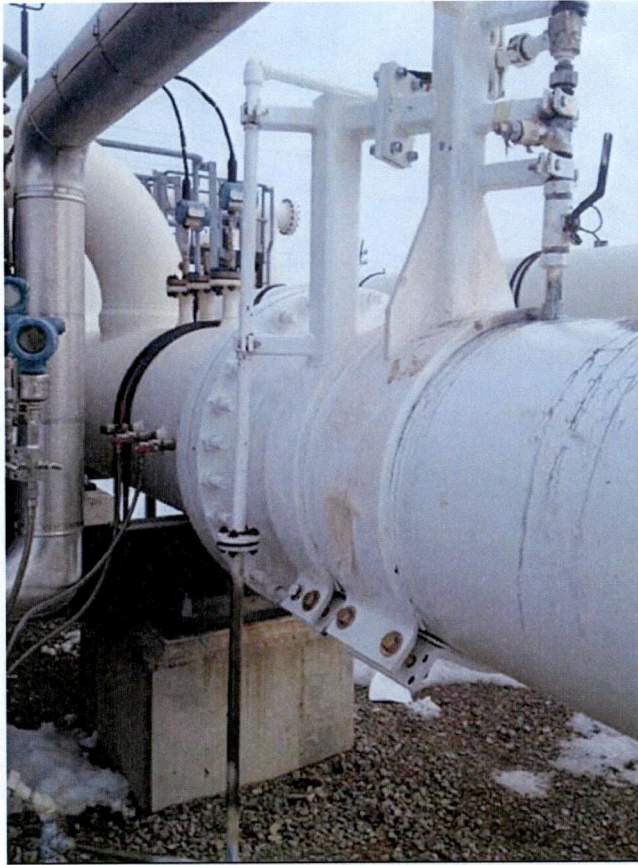
Figure 6: PSV-2206 assembly relocated to piping not exposed to vibration
