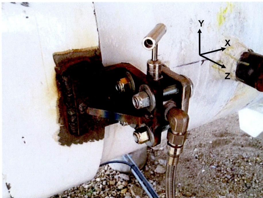
Figure 1: Braced PT-2207 root valve
