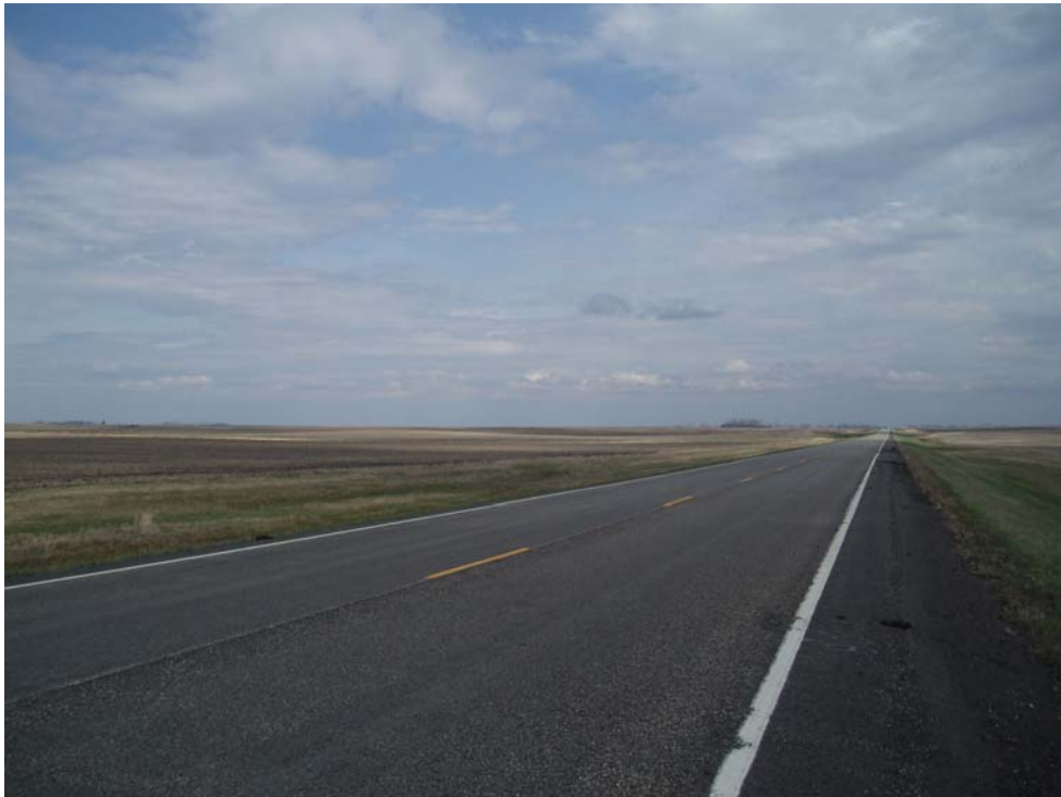
Proposed transmission line route running east to west in Section 36, Township 160 N and Range 60 W.
