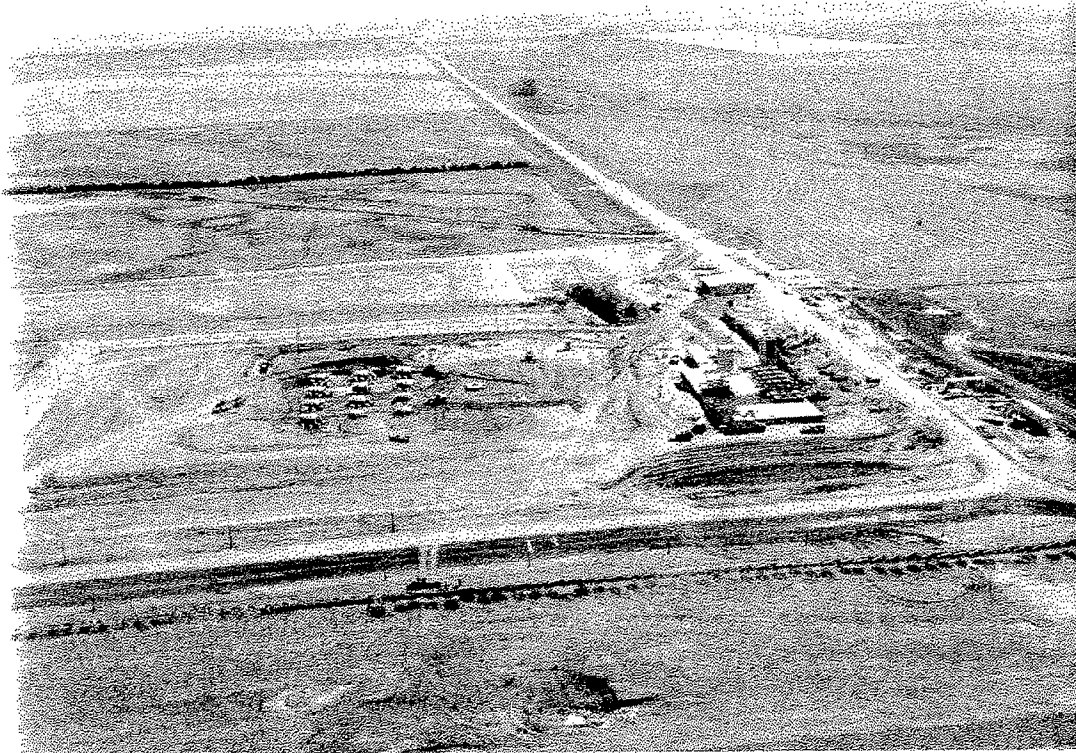
The Remote Sprint Launch Site #2 under construction in the fall of 1972. The tops of the Sprint Launchers are visible in the center of the picture. The building taking shape at the right was the Remote Launch Operations Building.
