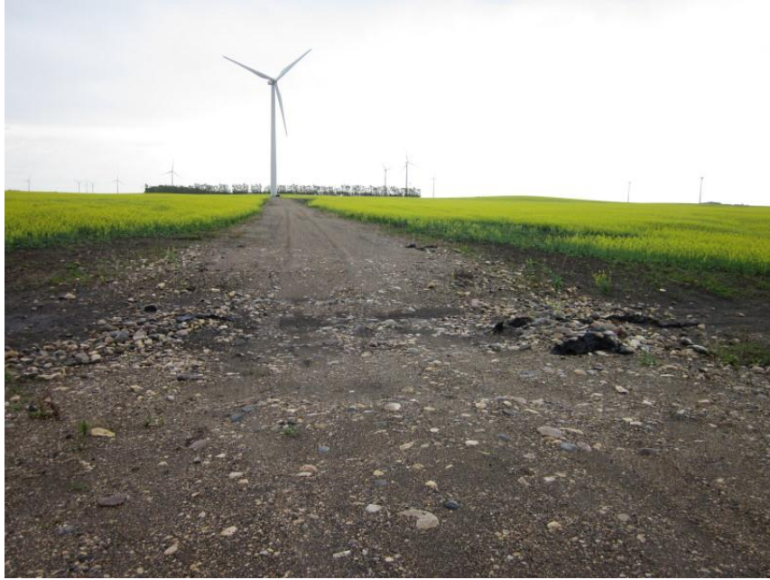
Photo 17. Direction: East. Texas crossing east of tower L2-11 between towers L2-11 and L2-12 (in distance). The crossing had been eroded to a deep and rough washout. A culvert would likely be better suited for the drainage at this particular crossing.
