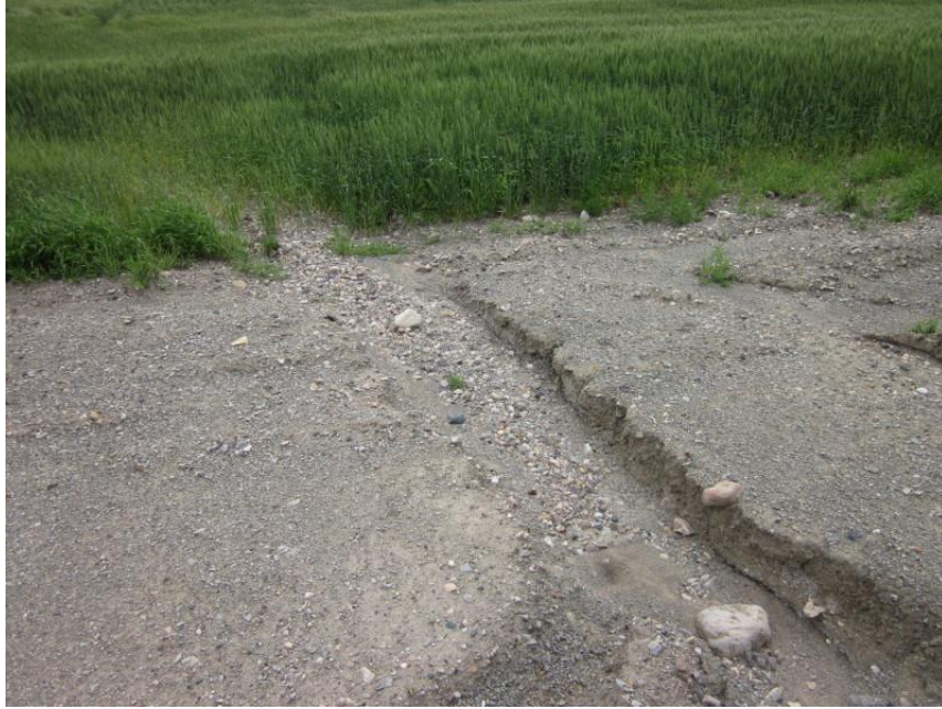
Photo 13. Direction: Southeast. Close-up of erosion on roadway, showing gravel being washed into adjacent field. NextEra stated that this problem has already been noted and will be repaired.
