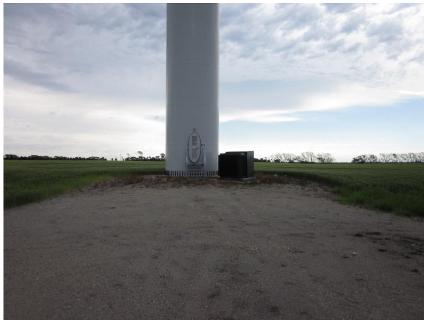
Photo 6. Direction: Northeast. Base of tower OT-17, showing an example of proper seasonal maintenance with annual weeds sprayed on the gravel pad. Note the surrounding crop was planted as close to the edge of the pad as possible by the landowner.
