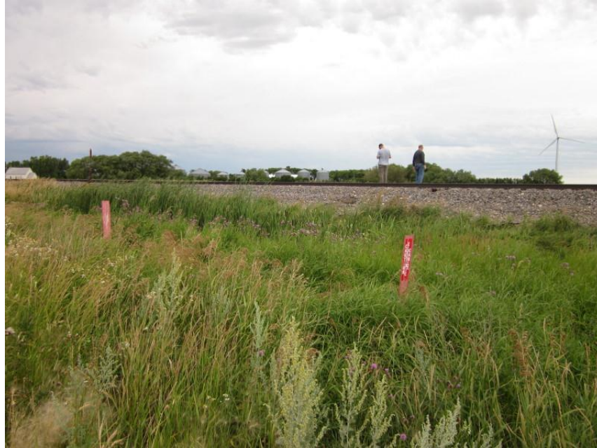
Photo 5. Direction: Northwest. Red markers indicate directional bore for utility line crossing underneath railroad tracks. The bore actually began and ended further out beyond the ditches in the adjacent fields. The railroad is a historical site (32CV121) and disturbance was avoided by boring. The vegetation in the ditches were typical wetland/mesic grassland vegetation that did not appear to have been disturbed, including reed canarygrass ( Phalaris arundinacea ), cattail ( Typha sp.), Canada thistle ( Cirsium arvense ), smooth brome ( Bromus inermis ), reedtop ( Agrostis stolonifera ), and Kentucky bluegrass ( Poa pratensis ).
