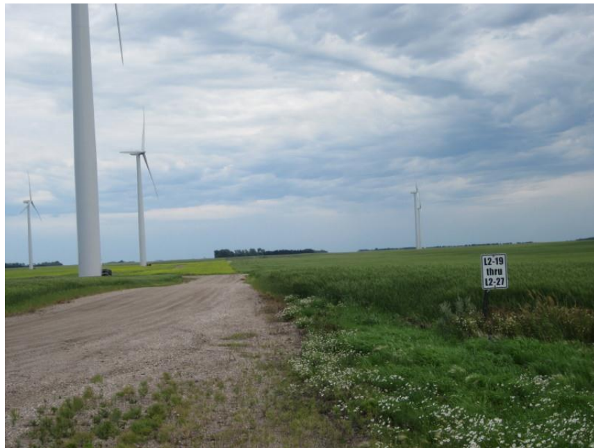
Photo 48. Direction: East. “No trespassing” sign missing from entrance to access road for towers L2-19 through L2-17.
