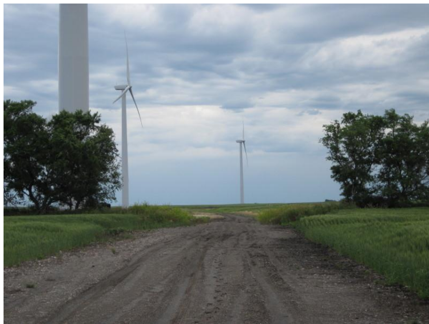
Photo 44. Direction: East. Access road between towers LD-55 and LD-54 showing where several Siberian elm trees had been removed from a planted tree row on the edge of a field. The cut was less than 50 feet in width, as required by the PSC.
