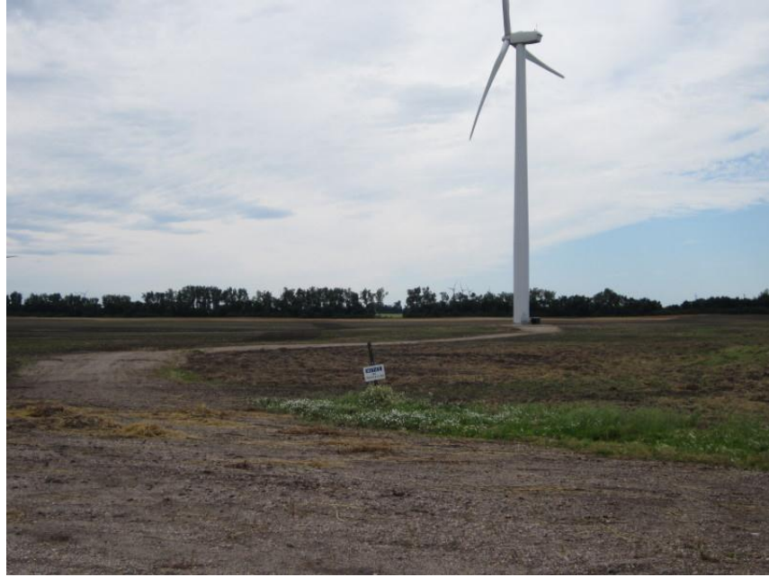
Photo 47. Direction: West. Sign missing on the entrance to the access road for tower L2-15.
