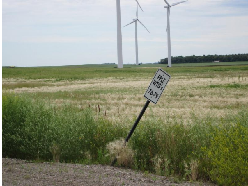
Photo 41. “No trespassing” sign was missing from post at entrance of access road to towers LD-76 to LD-79.
