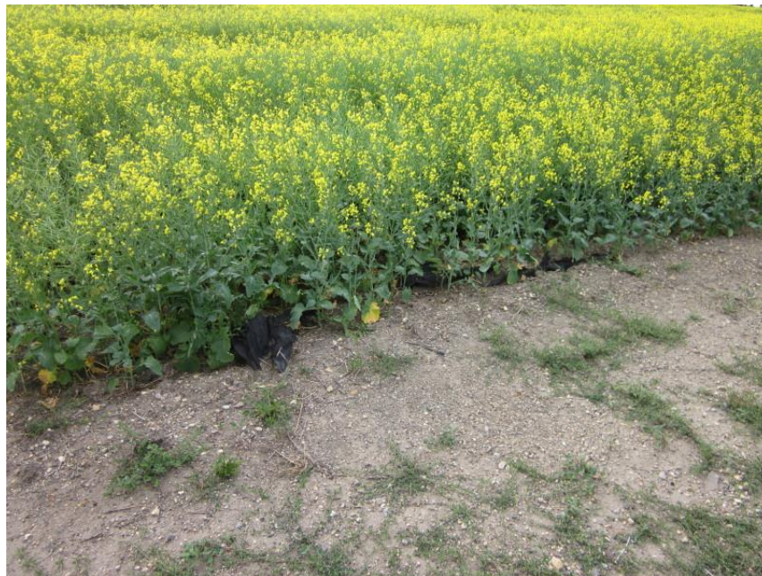
Photo 2. Close-up of Geotech fabric placed beneath gravel surfacing materials during construction was now visible in numerous locations. It reportedly gets washed out by rain and sometimes gets caught in farm implements.
