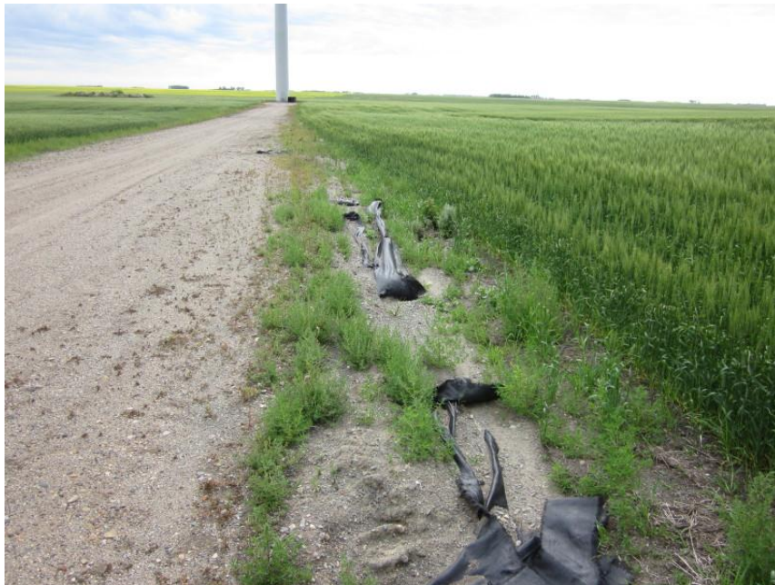
Photo 14. Direction: East. Erosion on edge of roadway between towers OT-14 and OT-15. The Geotech fabric was washed out on both sides of the road and the erosion extended partially across the roadway with sedimentation into adjacent fields.
