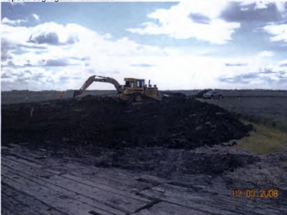
Topsoil segregation activities
