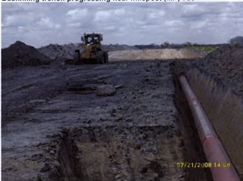
Backfilling trench progressing near milepost (MP) 786
