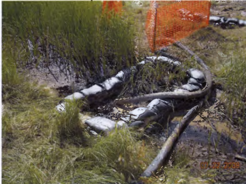
Containment and cleanup of minor drill mud release at S-792A (~milepost 792)
