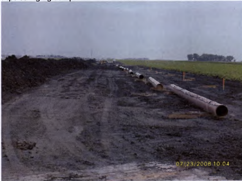
Backfilling trench progressing near milepost (MP) 786
