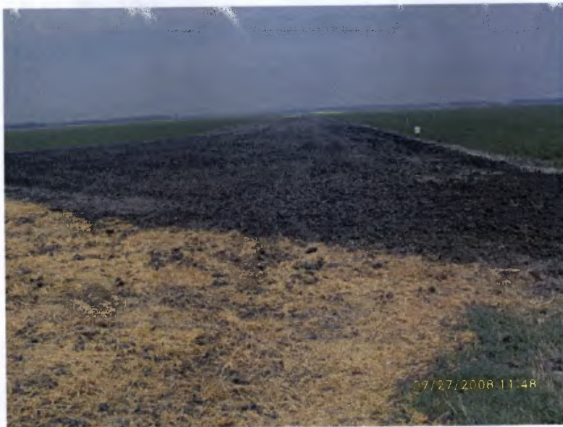
Tract 1098 (MP 779.5) decompaction completed and final grade established.
