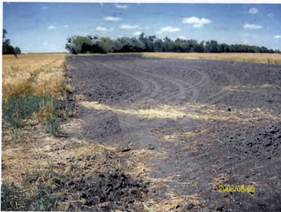
Restored right-of-way near MP 786.
