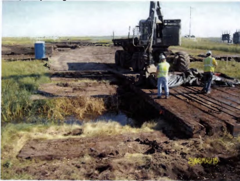
Temporary bridge removal
