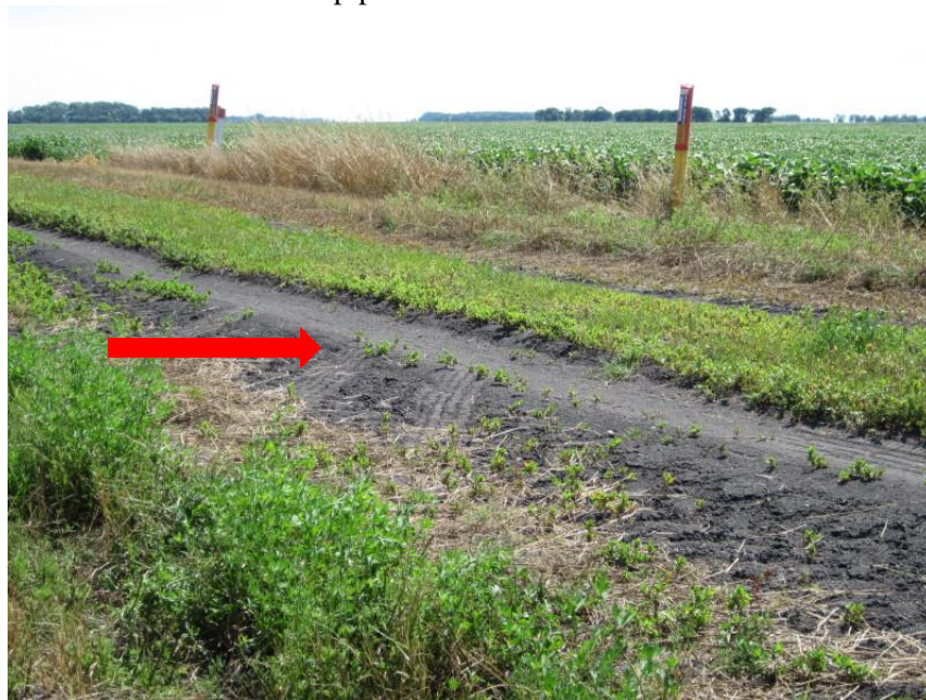
Photo 30. Direction: Southeast. Minimum maintenance portion of 104 th St NE to the southeast of Mile 781. The ditch vegetation and crops looked fine on either side, but there was a slight depression on the road from where the pipeline crossed (red arrow), which is difficult to see with this photo angle.
