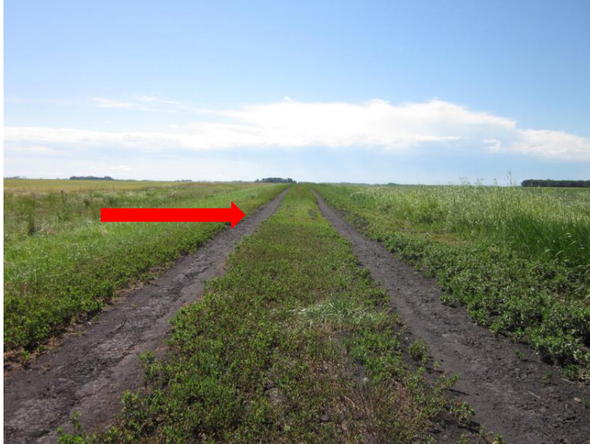
Photo 27. Direction: South. 148 th Ave NE just to the southeast of Mile 778. This road had been open cut and there was a slight depression where the pipeline route crossed (red arrow). It was not problematic for driving and there was no erosion, but the location should be monitored. The vegetation in the ditch had regrown completely and the crops adjacent to this area appeared to have no impacts.
