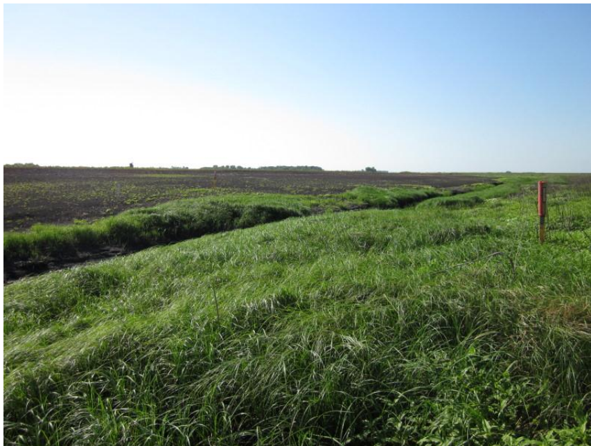
Photo 14. Direction: South. View of County Ditch 66-1 to the south, which diverges from the Red River within 0.5 miles north of this point. The crossing of the pipeline is indicated by the marker posts on either bank, and is just to the northwest of Mile 801. This crossing was directionally drilled underneath the ditch. There were no indications of vegetation disturbance or erosion problems.
