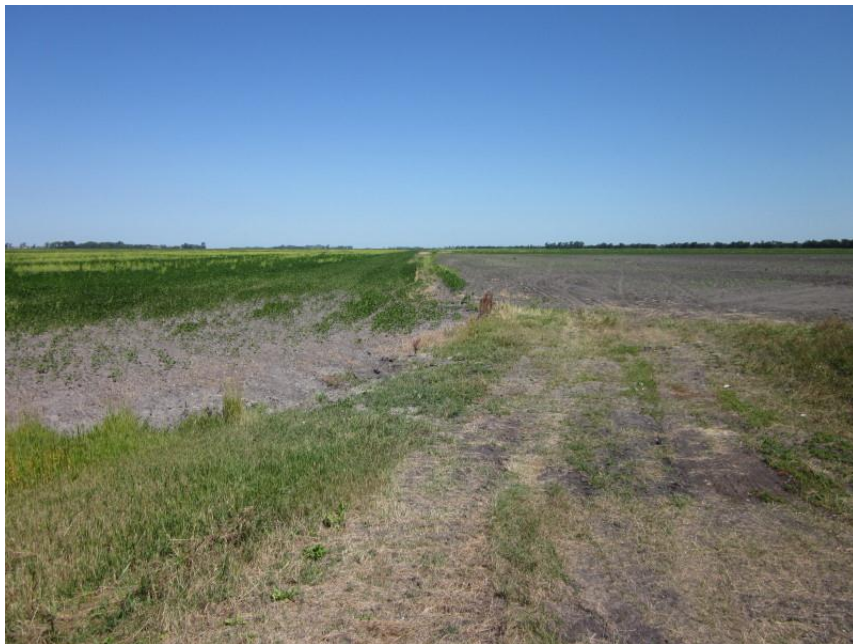
Photo 18. Direction: North. Location of temporary access road, going straight north from 109 th St NE to approximately Mile 773.9 on the pipeline route. There was no indication of the access road. The cropland and road ditches of 109 th St NE had been completely restored to prior condition.
