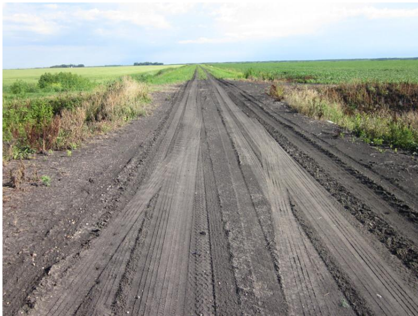
Photo 8. Direction: North. Minimum maintenance section line road was restored (161 st Ave NE) and showed no signs of construction. This was to the southeast of Mile 797.
