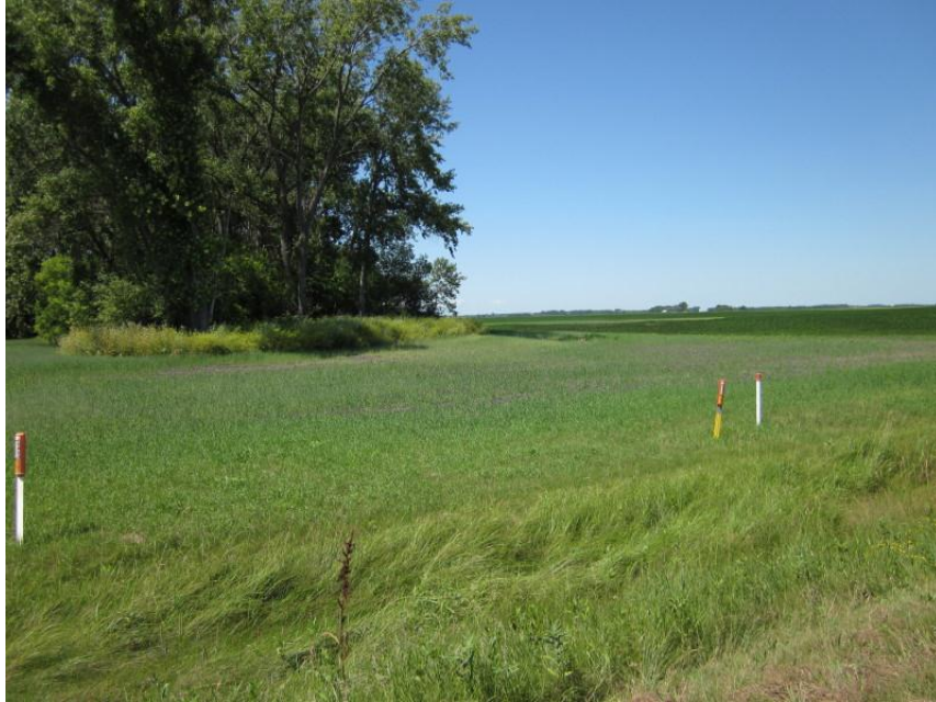
Photo 35. Direction: Northwest. Along 155 th Ave NE between Miles 788 and 789, showing route of pipeline where the workspace width was reduced to less than 50ft to minimize the number of trees removed from tree rows surrounding another farmyard.
