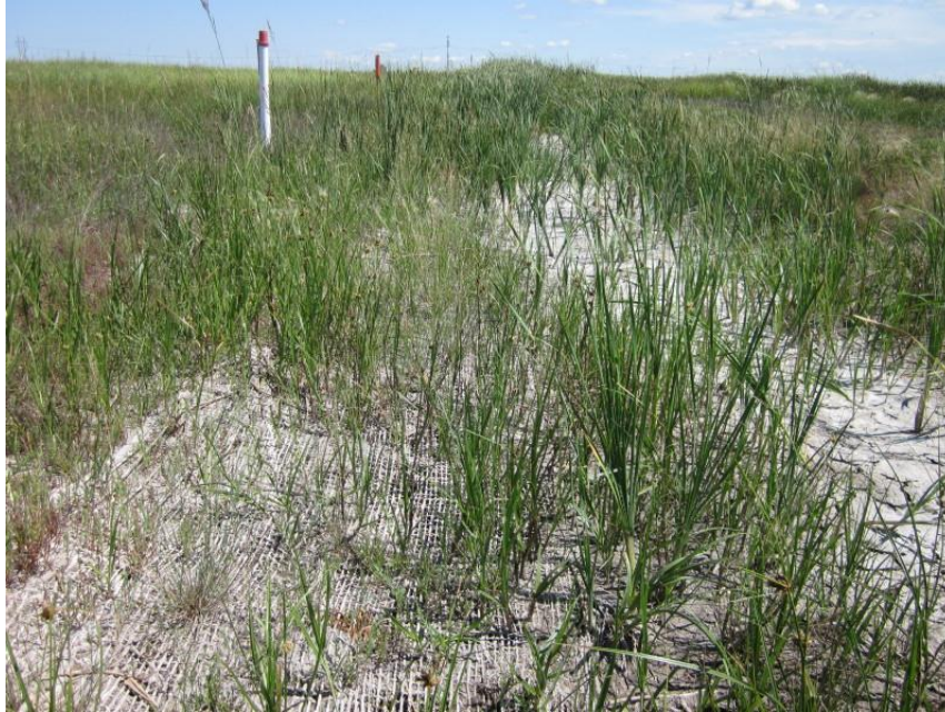
Photo 37. Direction: East. Ditch along minimum maintenance portion of 97 th St NE between Miles 790 and 791, within the wetlands surrounding Juhl National WMA. Pipeline route is marked by the posts on the left. Jute netting was in place in the ditch to stabilize soils and was functioning well. New vegetation was growing through the netting, including many native species such as prairie cordgrass ( Spartina pectinata ) and cattails ( Typha sp.) and the non-native but common grass quackgrass ( Agropyron repens ).
