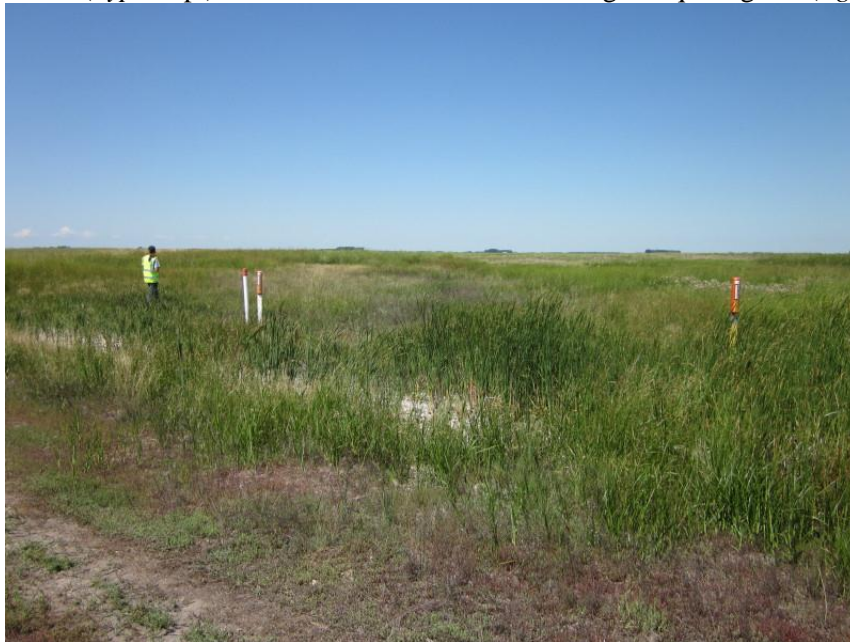
Photo 37. Direction: East. Ditch along minimum maintenance portion of 97 th St NE between Miles 790 and 791, within the wetlands surrounding Juhl National WMA. Pipeline route is marked by the posts on the left. Jute netting was in place in the ditch to stabilize soils and was functioning well. New vegetation was growing through the netting, including many native species such as prairie cordgrass ( Spartina pectinata ) and cattails ( Typha sp.) and the non-native but common grass quackgrass ( Agropyron repens ).
