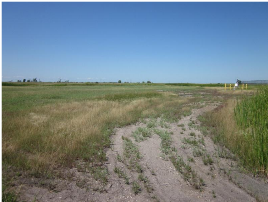
Photo 40. Direction: Northwest. West side of Joliette pumping station grounds near Mile 792 where the pipeline veers south to cross State Highway 5. Pipeline runs to the south of above-ground valve visible on right.
