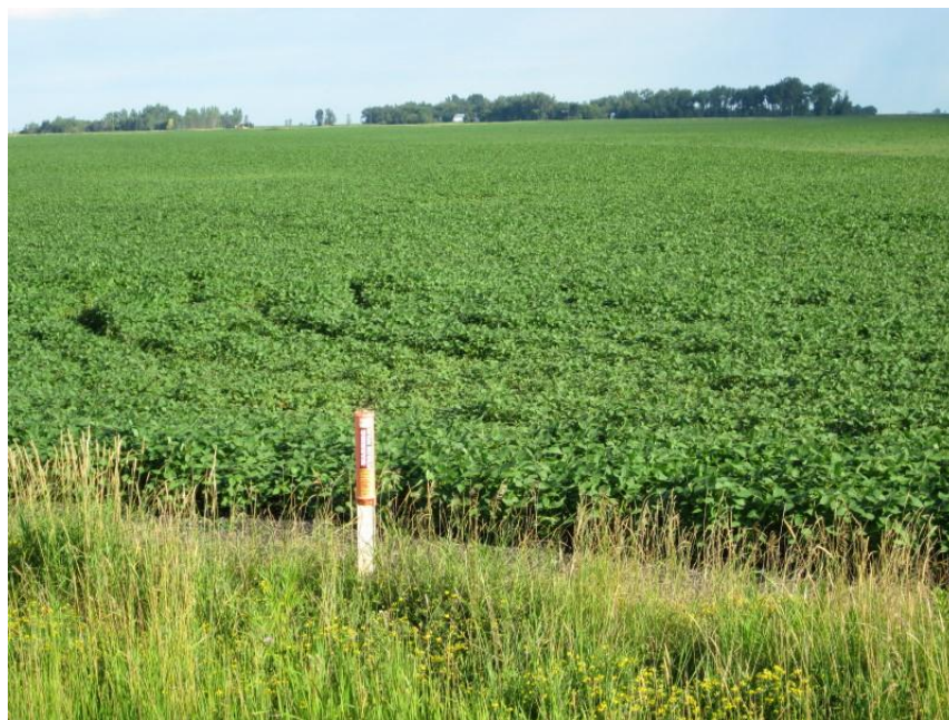
Photo 4. Direction: Northwest. Ditch and field to the northwest of 93 rd Street NE at Mile 796.4. The road had been directionally bored underneath, denoted by pipeline marker in foreground. There appeared to be a slight depression and stunted, slightly yellowed crop at the end of the bore in the field.
