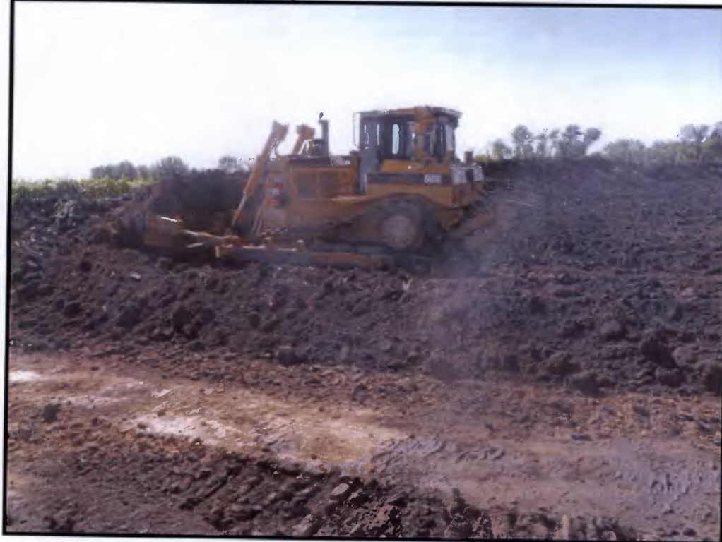
Topsoil segregation activity in agricultural area
