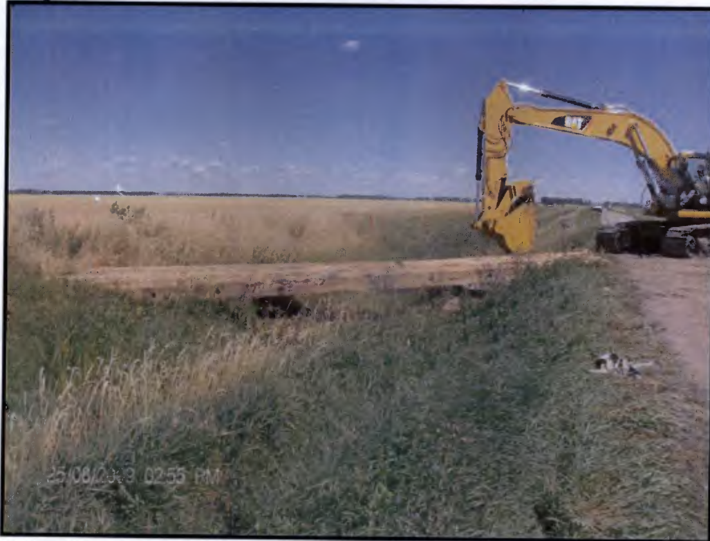
Topsoil segregation activity in agricultural area
