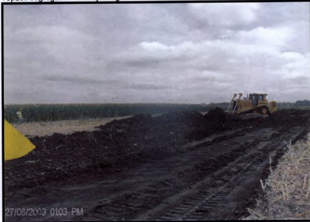
Topsoil segregation activity in agricultural area
