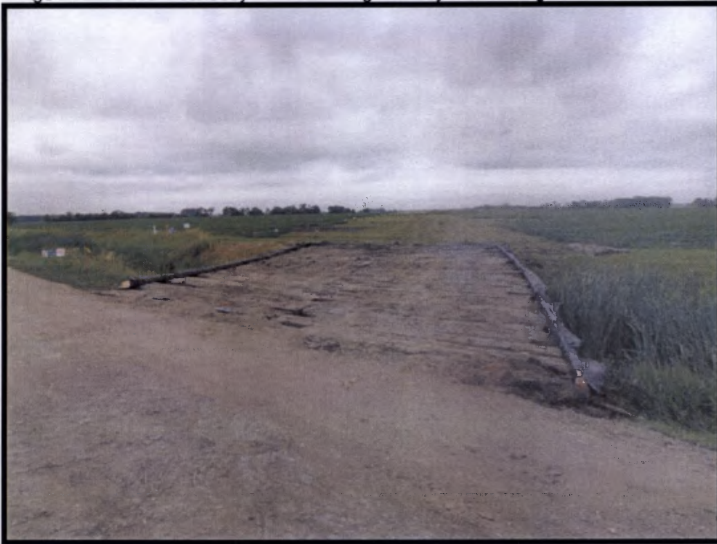
Bridge installed over waterbody with cleared right-of-way in the background
