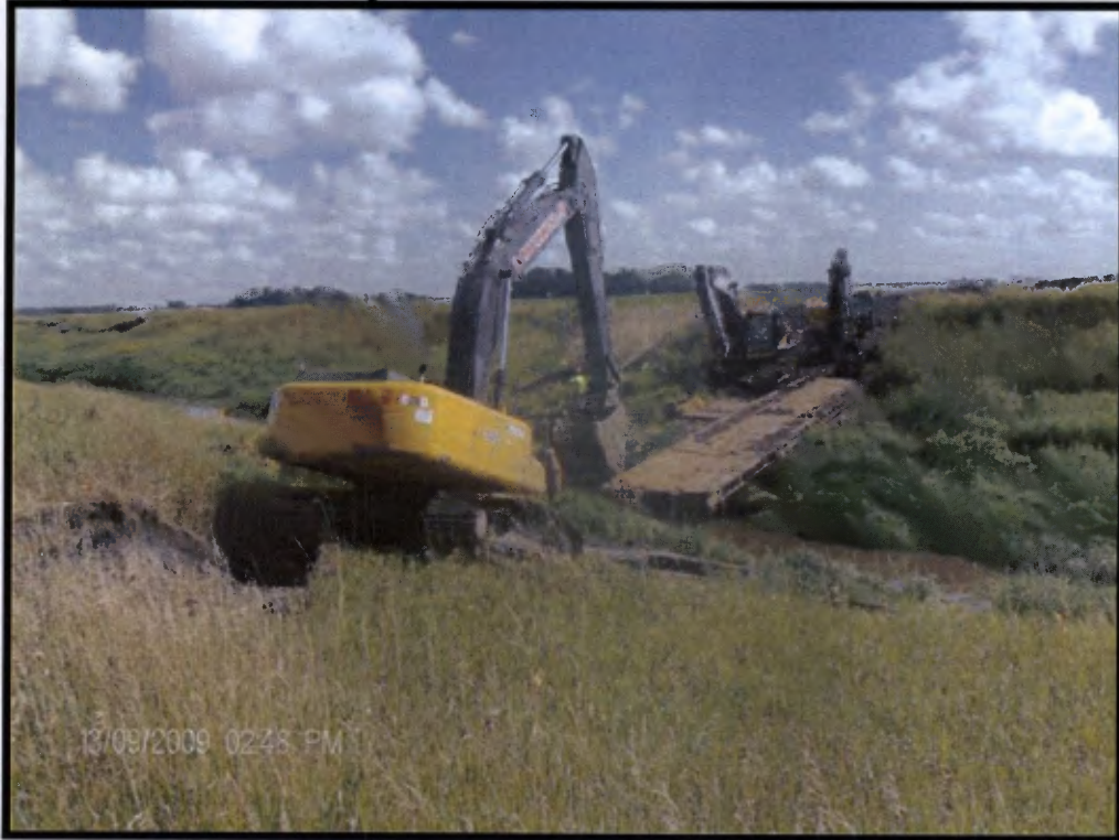
Bridge installation at the Tongue River "cutoff"
