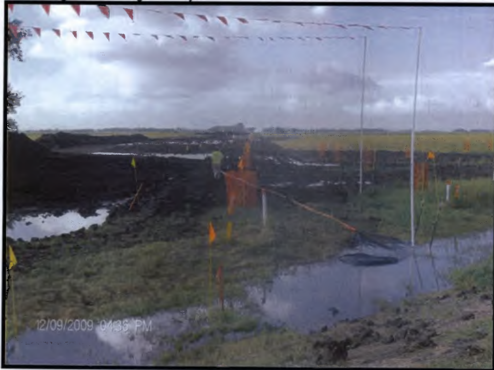
Horizontal directional drill equipment set up near Pembina River
