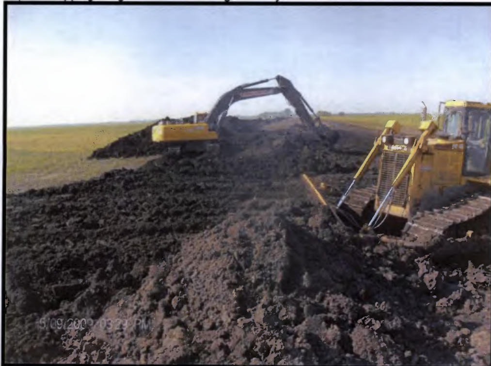
Topsoil stripping in agricultural area of right-of-way
