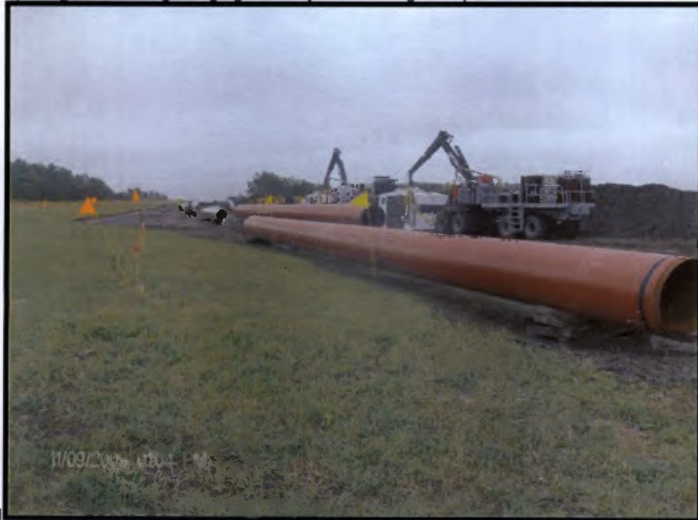
Pipe segments strung along right-of-way with welding units parked behind
