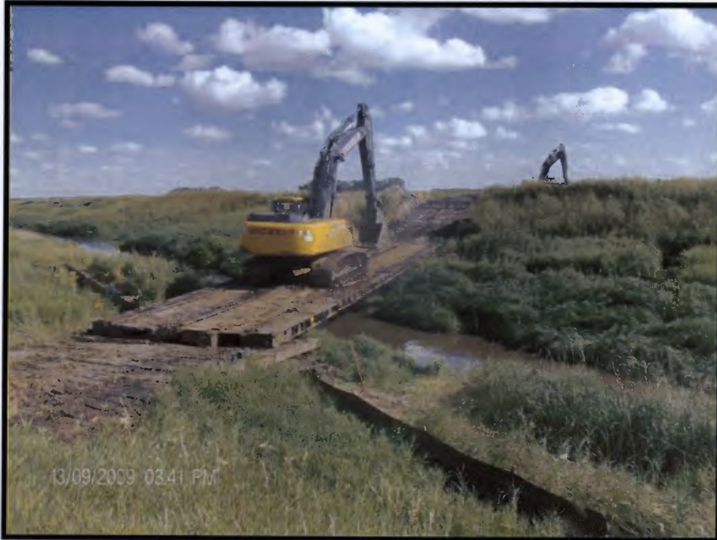
Dewatering of flooded right-of-way area
