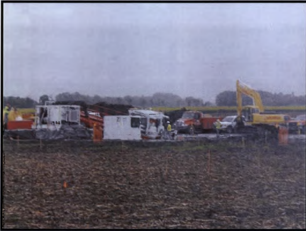
Pipe segments strung along right-of-way with welding units parked behind
