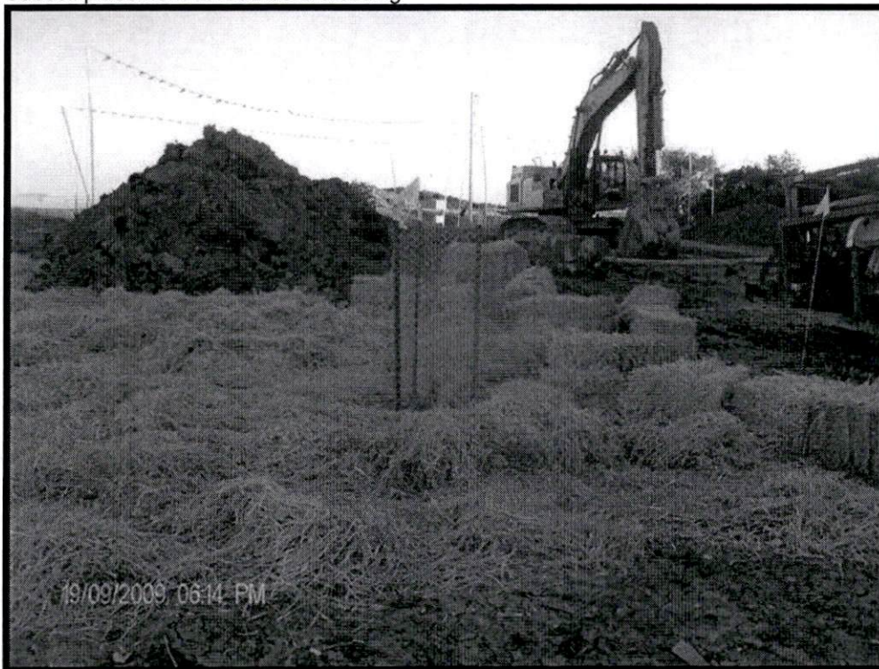
Subsoil placement at road bore crossing
