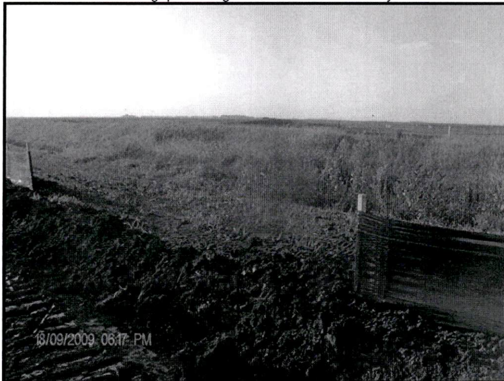
Silt fence installed with gap for bridge installation at waterbody
