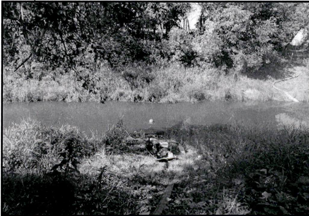
Intake hose suspended off the bottom of waterbody s-886a with a intake screen, pump in secondary containment
