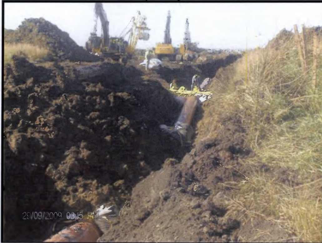
Installation of trench breaker at waterbody crossing
