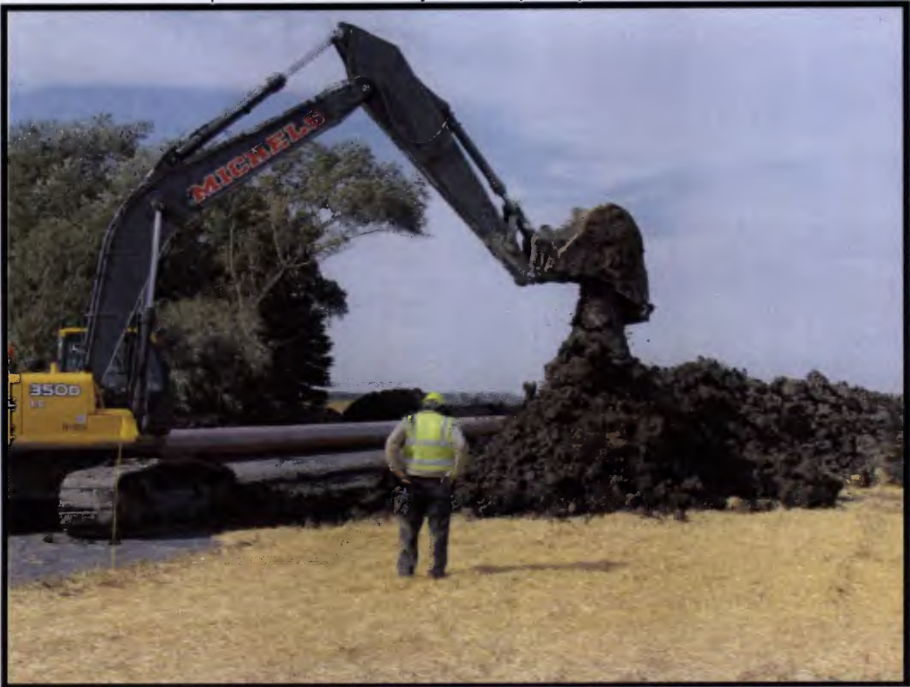
Trench excavation placed on mulch layer for topsoil protection
