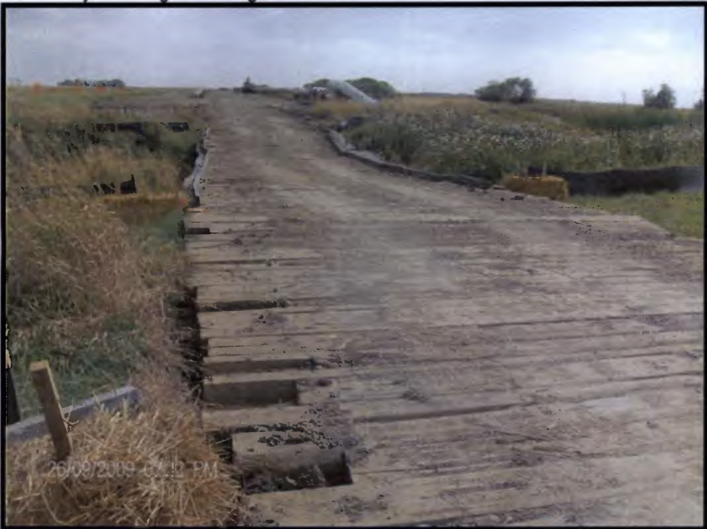
Waterbody crossing with bridge and erosion controls
