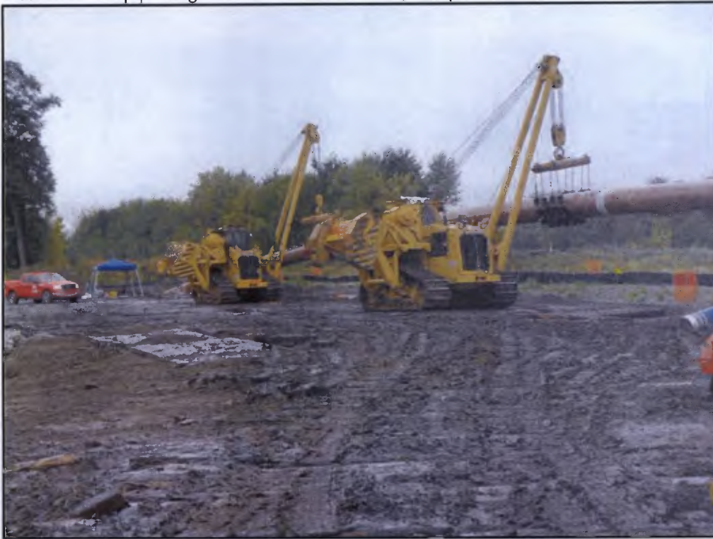
Mats for access road down to south side of the Red River of the North crossing
