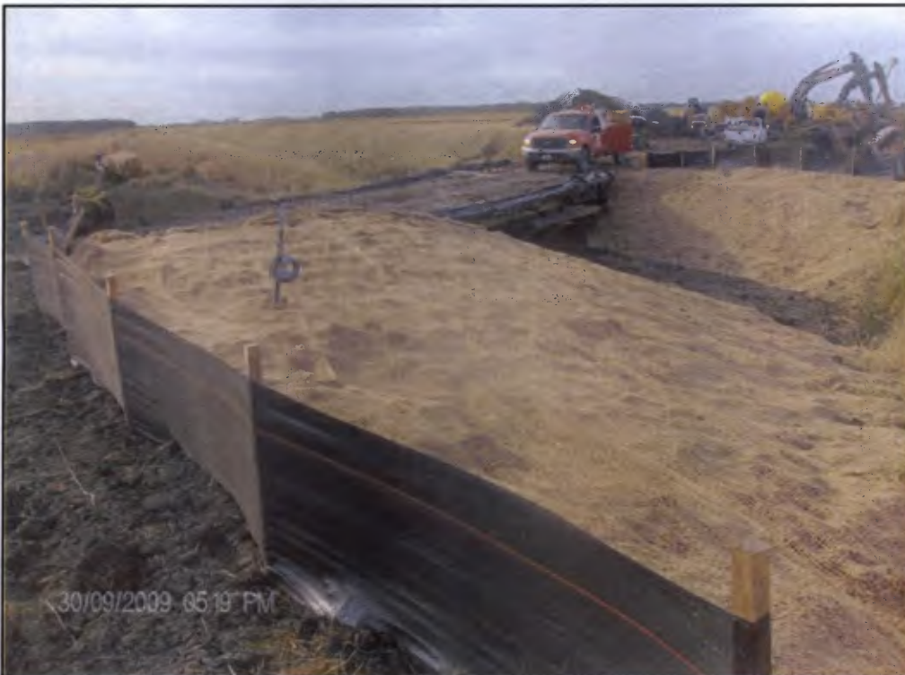
Stabilization and erosion control installation at S-778a
