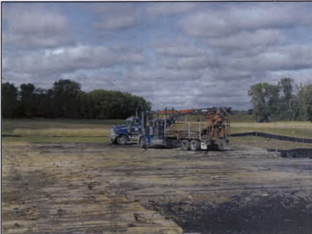
Mats for access road down to south side of the Red River of the North crossing
