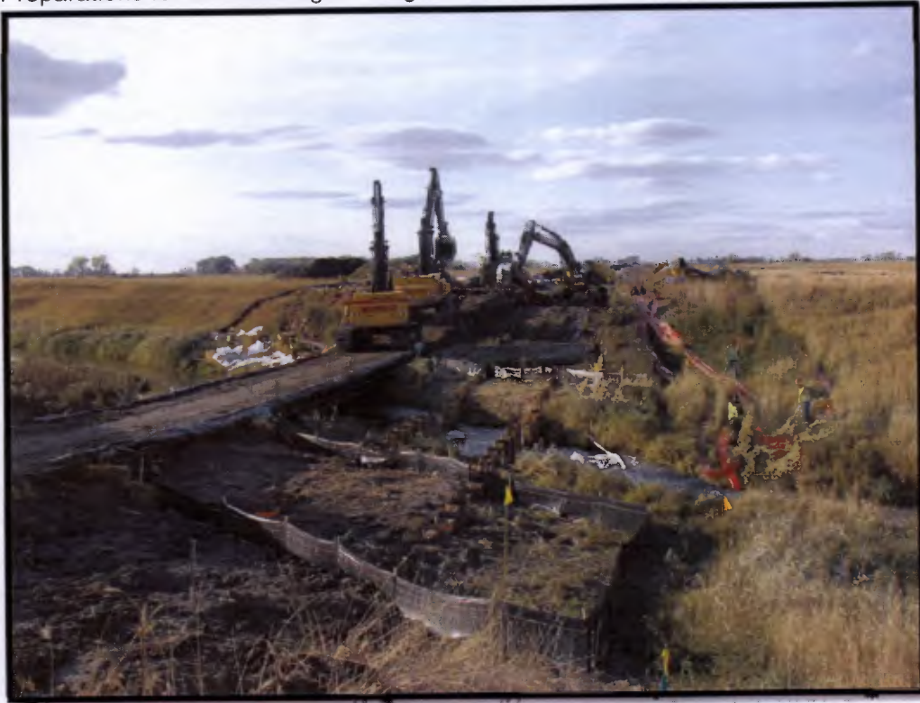
The HDD rig conducting the crossing of the Red River of the North
