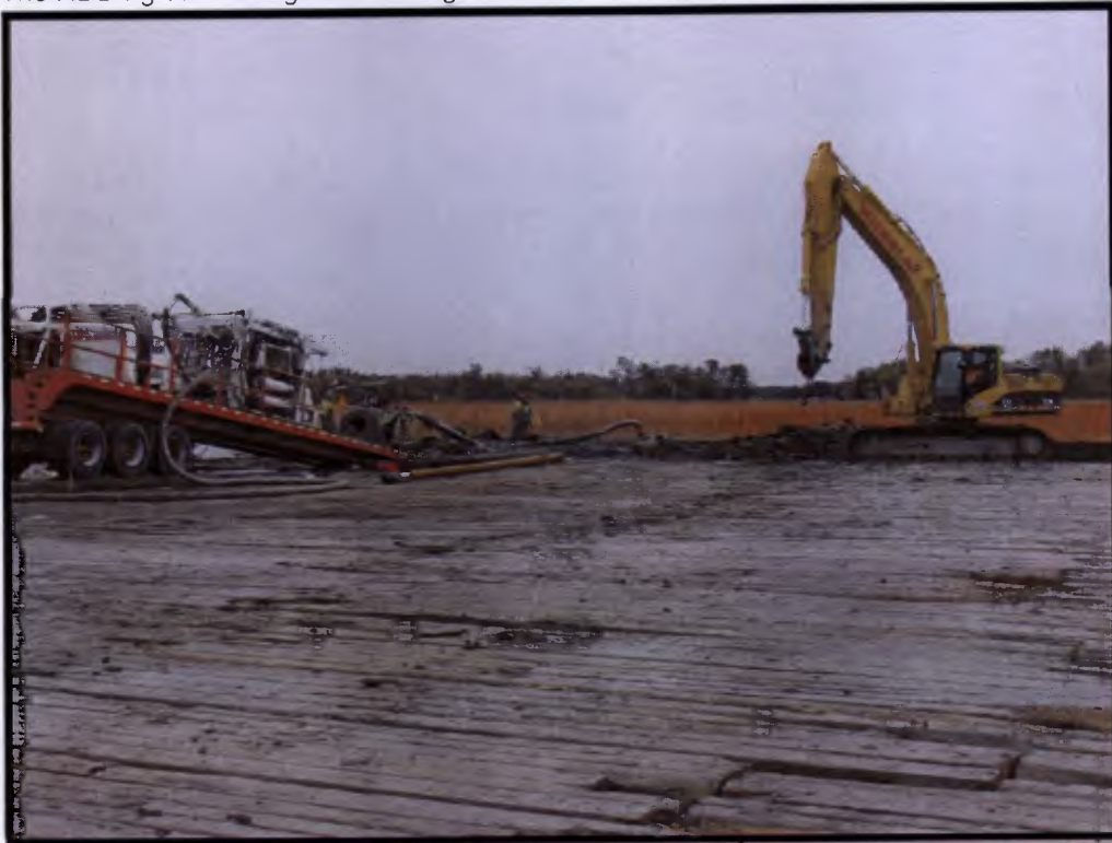
The HDD rig conducting the crossing of the Red River of the North
