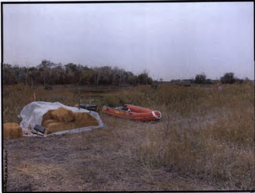
Materials placed at Red River of the North banks for potential drilling mud release response
