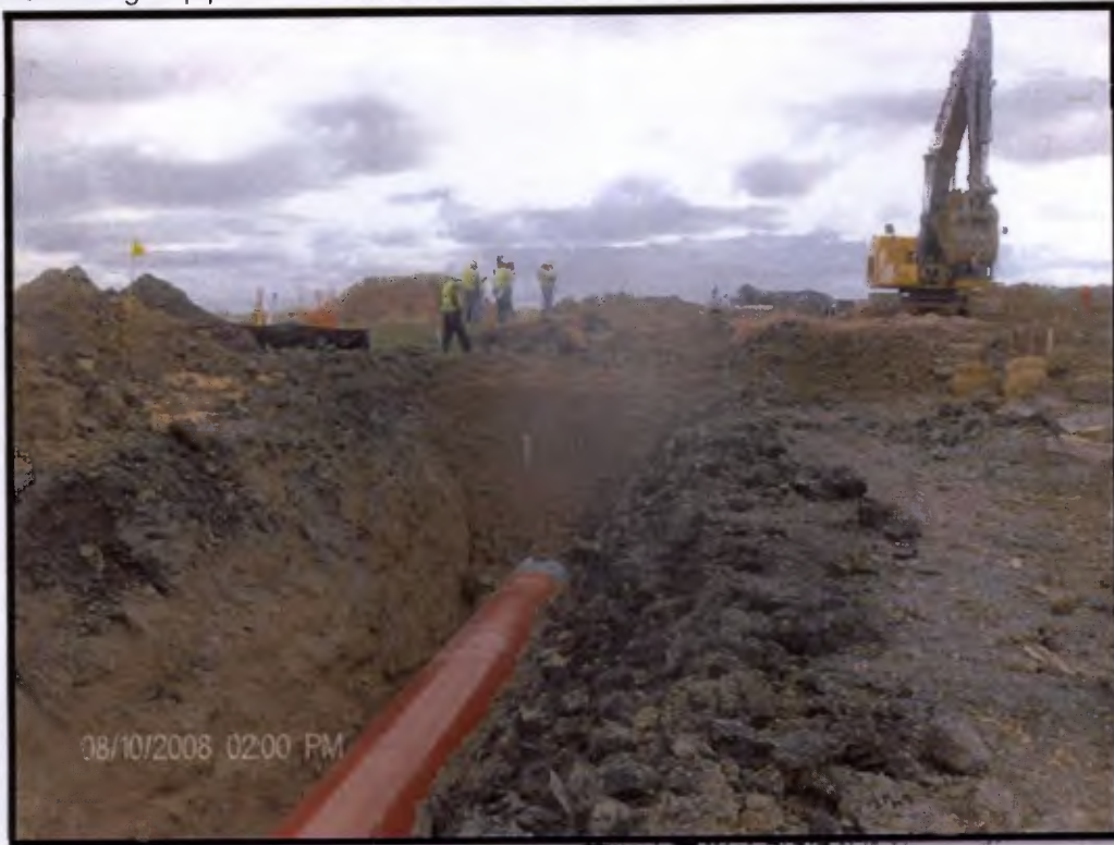
Backfilling of pipeline at 100 th Street NE
