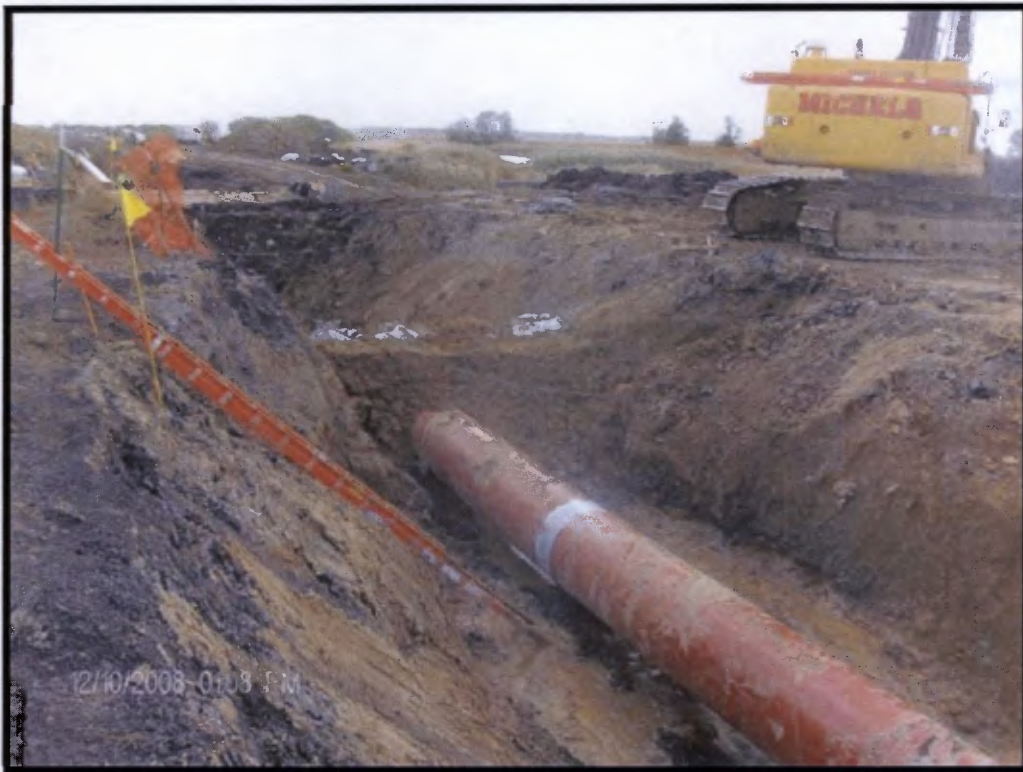
Trench breaker installation near wetland w-782b
