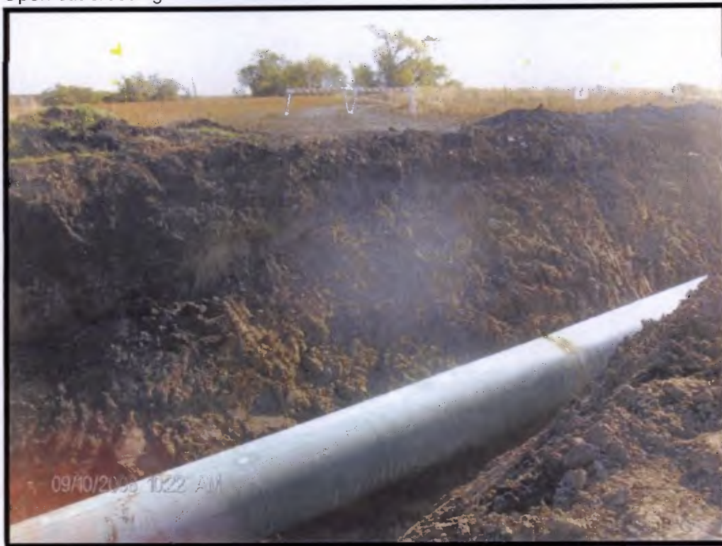
Open cut crossing of 103 rd Street NE
