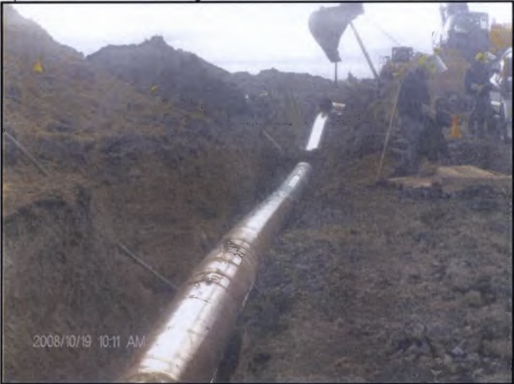
Pipeline installation and welding activities
