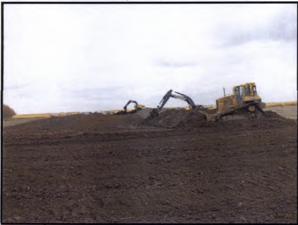
Restoration of topsoil across the right-of-way
