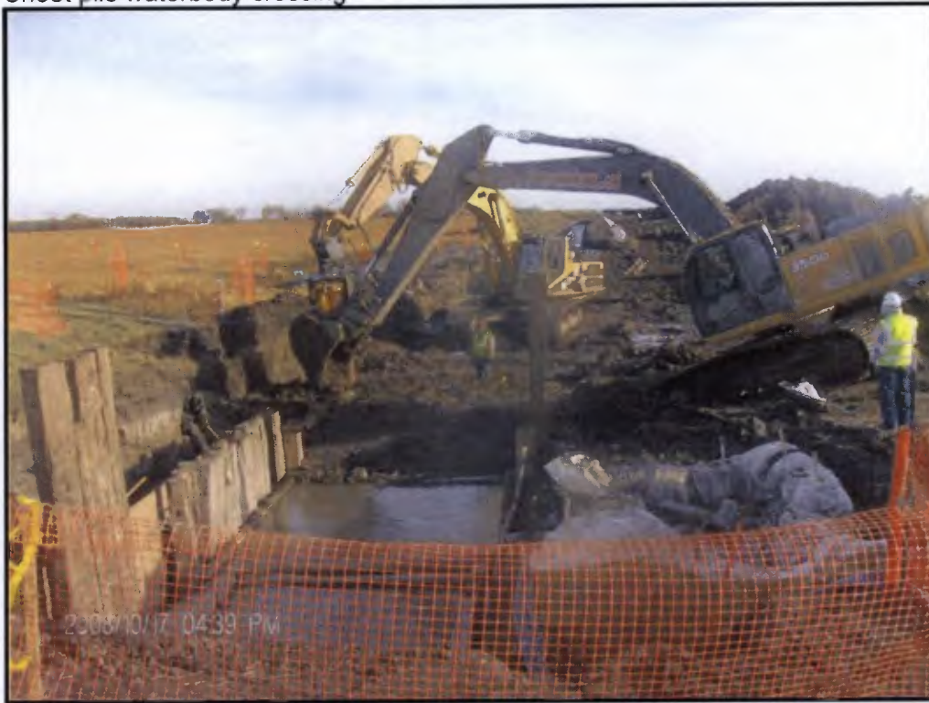
Sheet pile waterbody crossing
