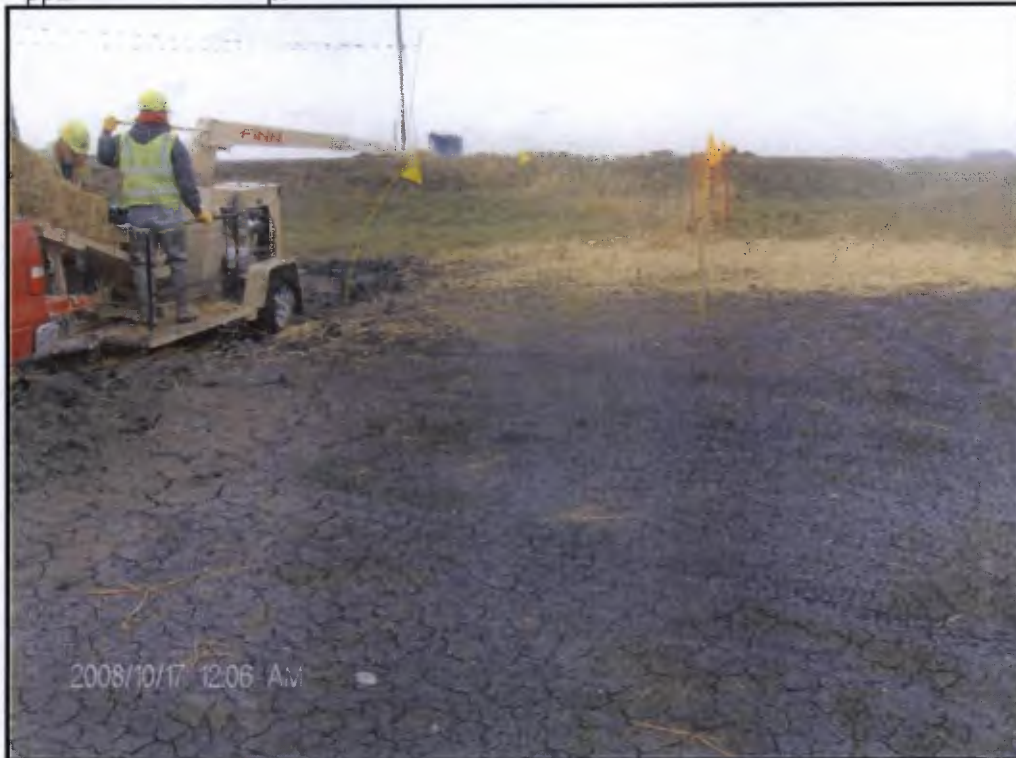
Application of mulch prior to trench excavation
