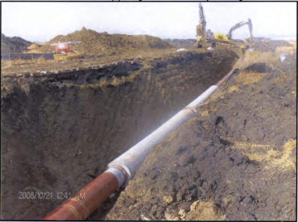
Installation of concrete coated pipe segment at waterbody crossing
