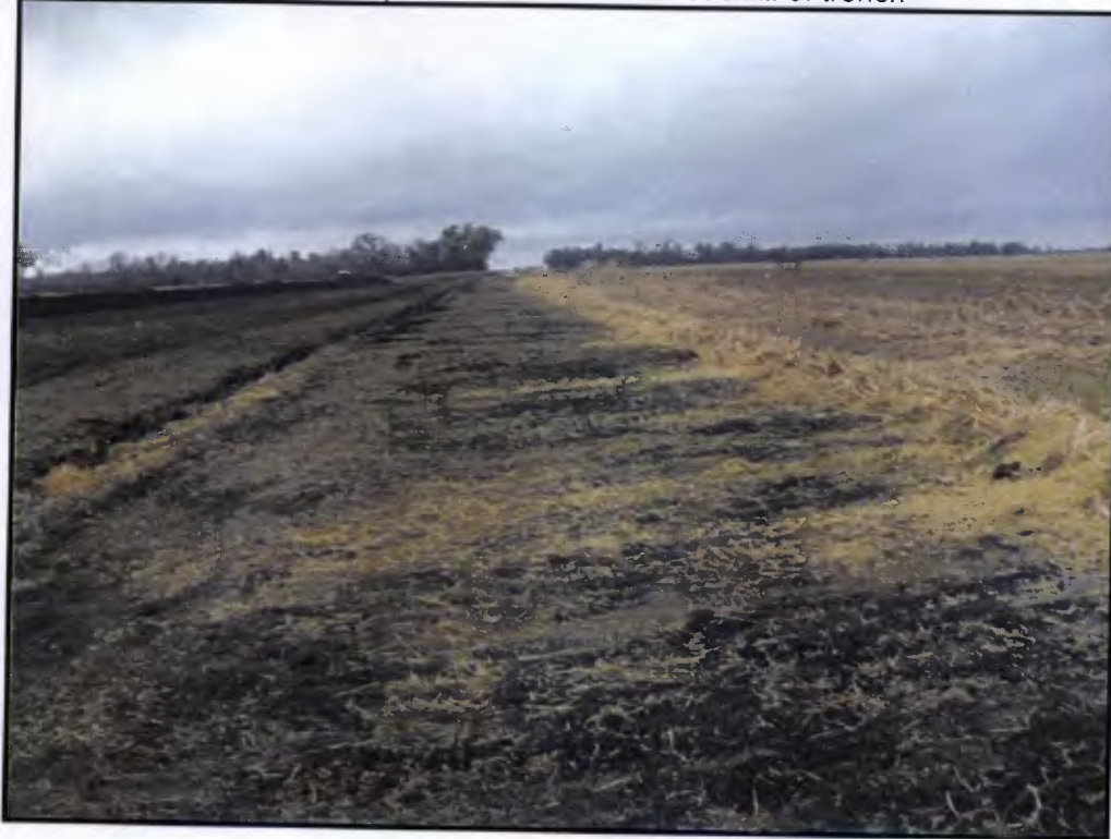
Clean-up of trench subsoil placed on mulch after backfill of trench
