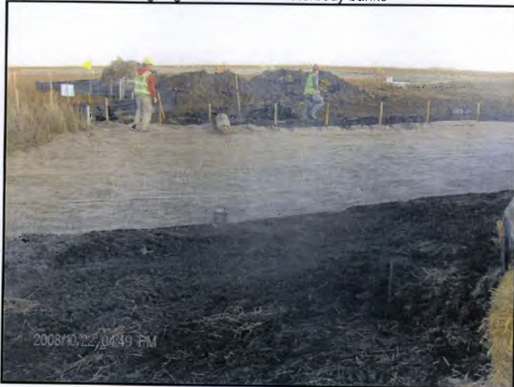
Topsoil backfill and ongoing stabilization of waterbody banks
