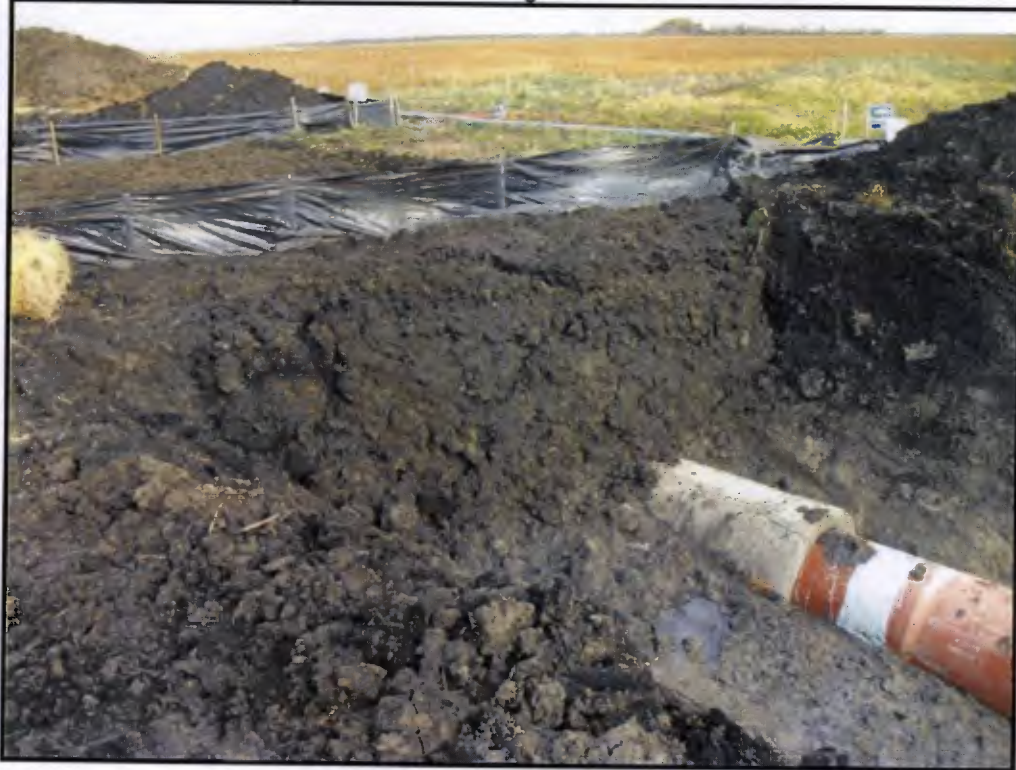
Lowering-in and tie-in of pipeline
