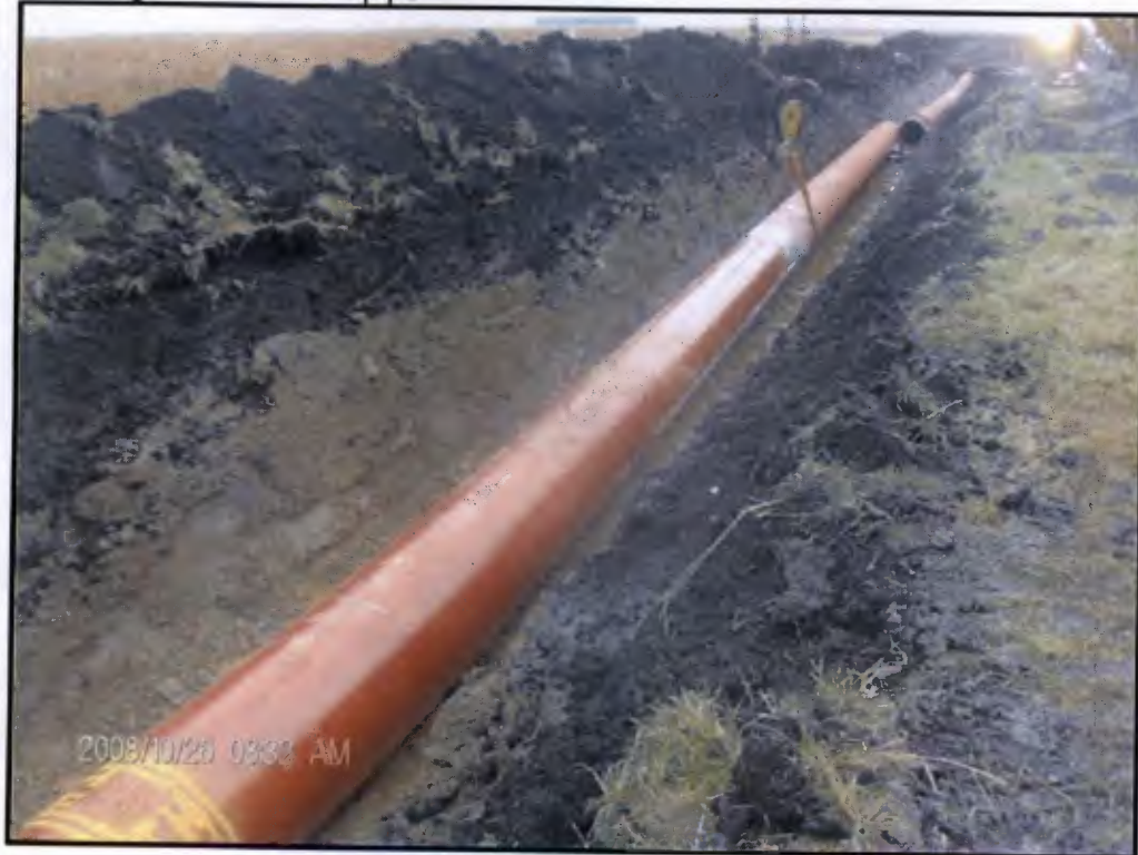
Lowering-in and tie-in of pipeline
