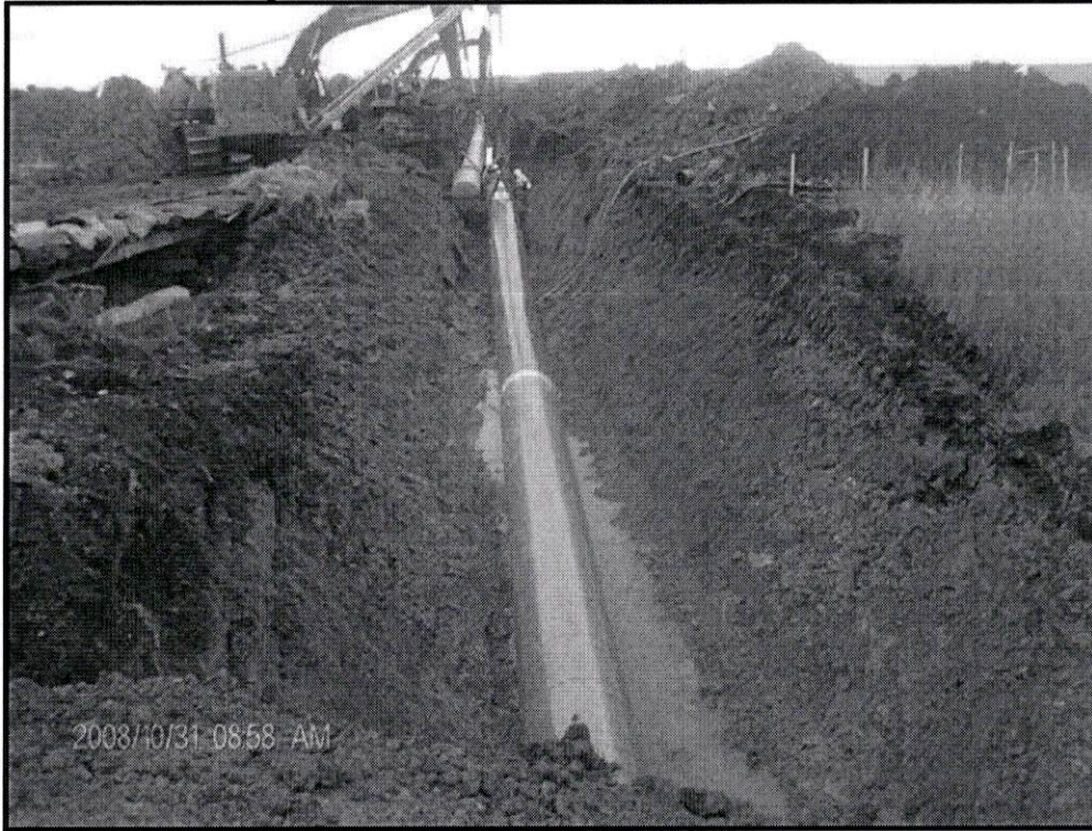
Trench box removal following completion of road bore crossing
