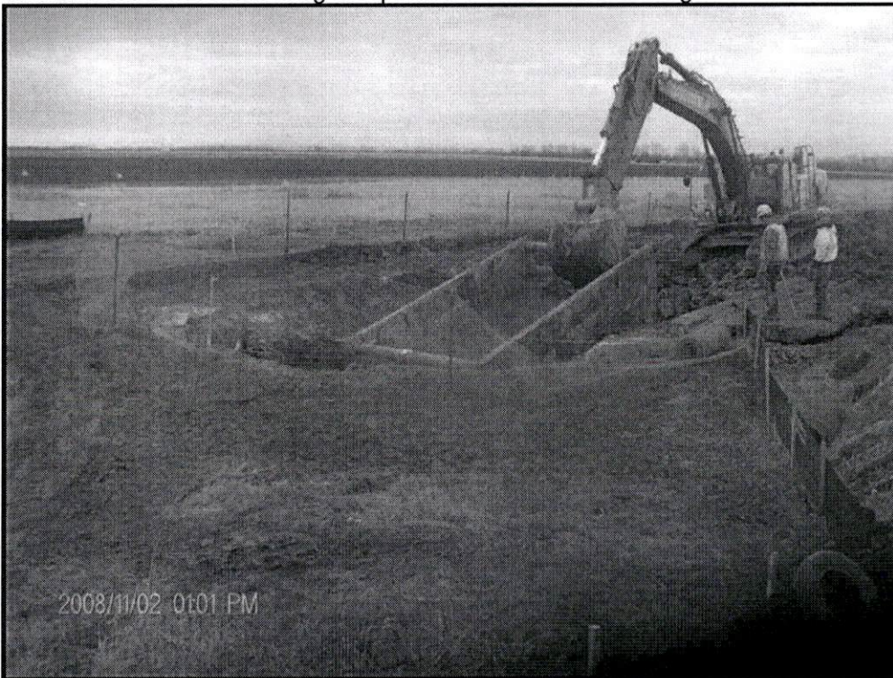
Trench box removal following completion of road bore crossing
